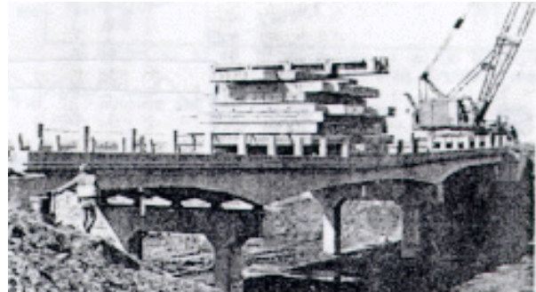
Figure 12 - Load test of Canadian t-beam bridge. (Picture Courtesy of NRC Research Press)
