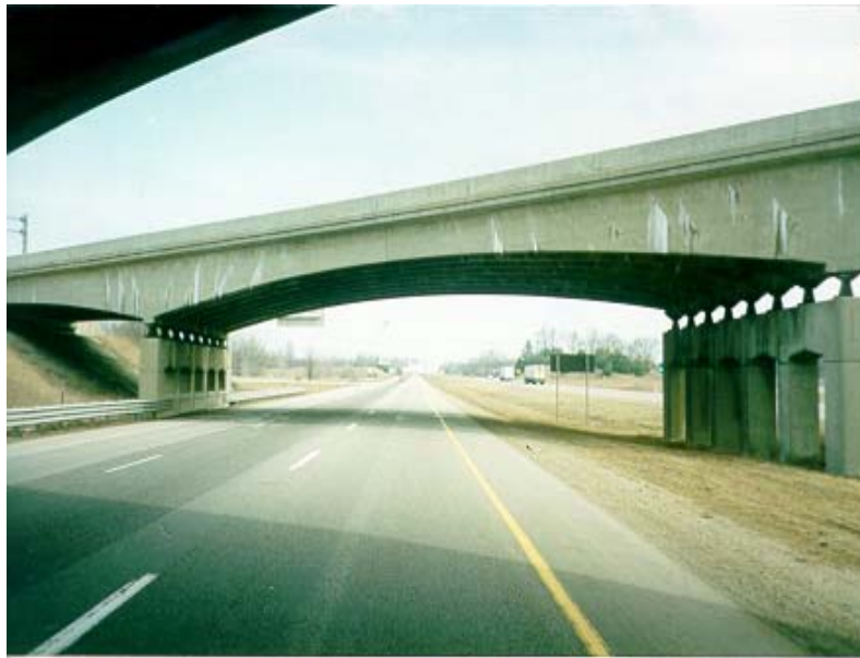
Figure 1- Variable Depth T-Beam Bridge
