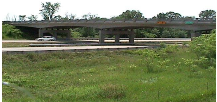
Figure 13 - Jones Road over I-96.
