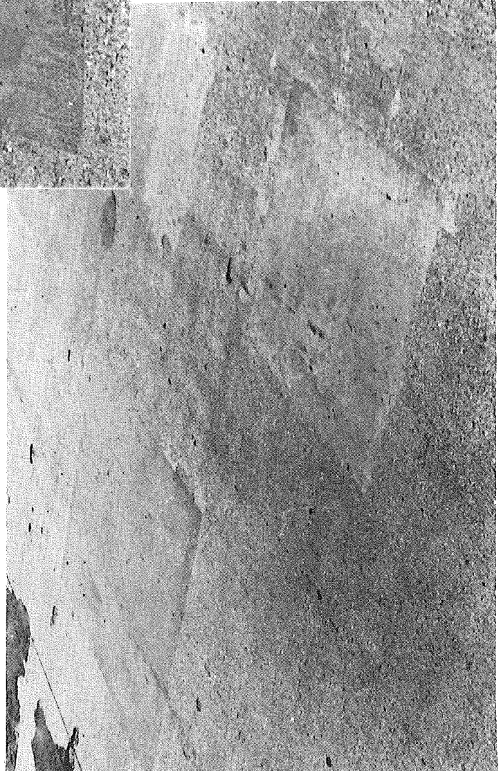
Figure 5. Patches placed 7-26-66 in Paterson St. bridge over Kalamazoo River in Kalamazoo. Over-all view shows three patches in north half of east end span near pier three. Close-up shows largest patch, about three-feet square, and sawed perimeter.
