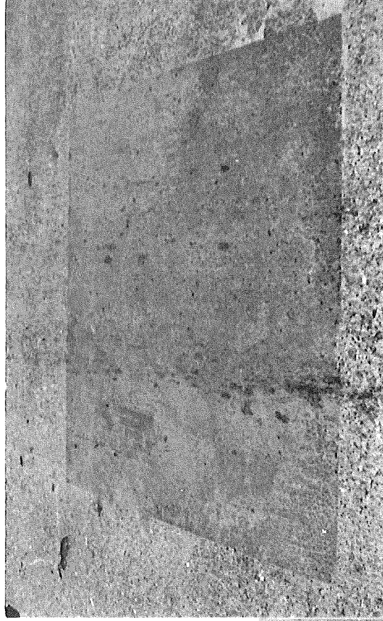
Figure 5. Patches placed 7-26-66 in Paterson St. bridge over Kalamazoo River in Kalamazoo. Over-all view shows three patches in north half of east end span near pier three. Close-up shows largest patch, about three-feet square, and sawed perimeter.
