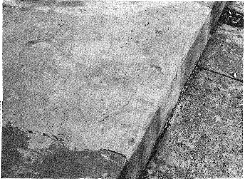
Figure 2. Close-up of patch placed 4-29-66 in front of Gladmer Theater showing shrinkage cracks near corner. Second view shows original patch and additional ones placed in September, 1966, by Lansing DPW.
