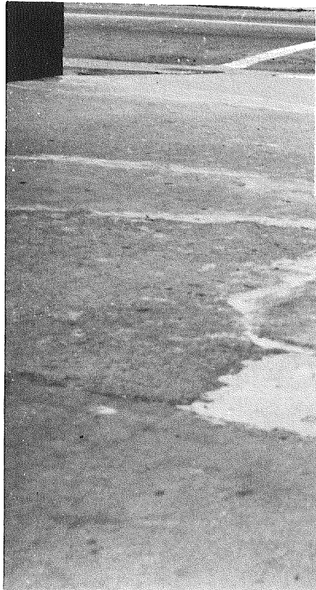
Figure 2. Close-up of patch placed 4-29-66 in front of Gladmer Theater showing shrinkage cracks near corner. Second view shows original patch and additional ones placed in September, 1966, by Lansing DPW.
