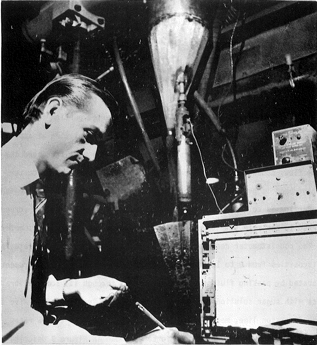
Figure 8. Consistometer and density gauge connected to pilot plant medium circulation system.
