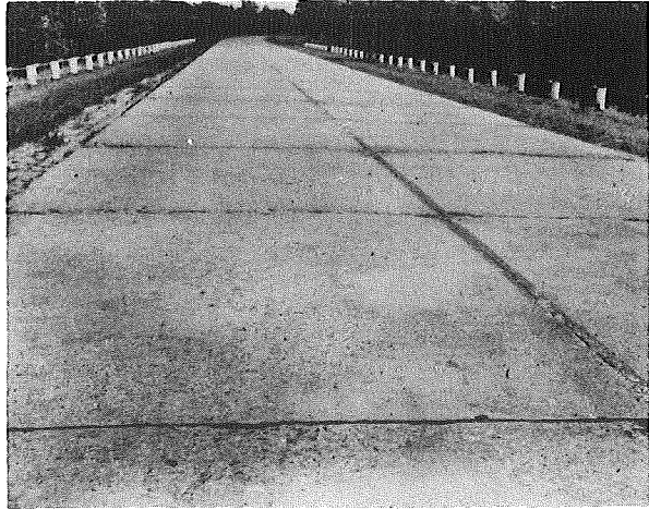
Section 7B Station 124+00 Looking South
