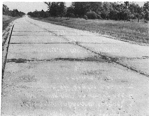
Section 6C Station 106+00 Looking South
