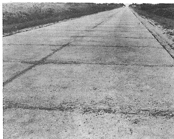
Section 7D Station 130+40 Looking North
