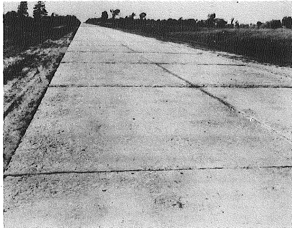
Section 8B Station 141+00 Looking North
