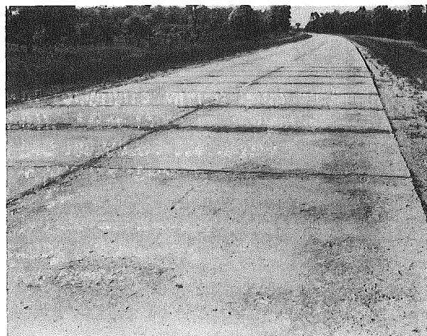
Section 6D Station 106+30 Looking North
