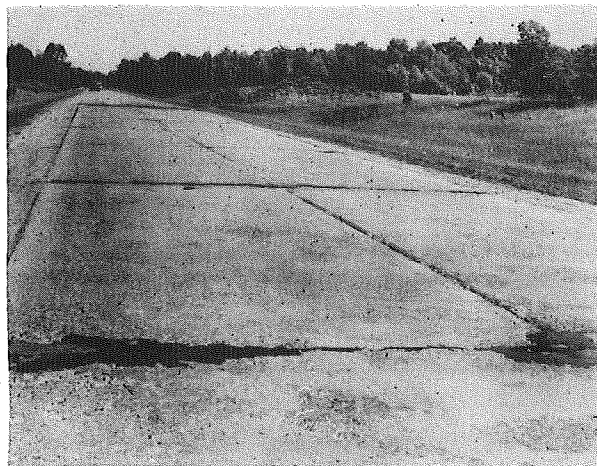
Section 8A Station 138+30 Looking South
