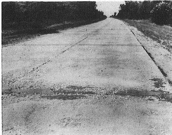
Section 7A Station 114+00 Looking North
