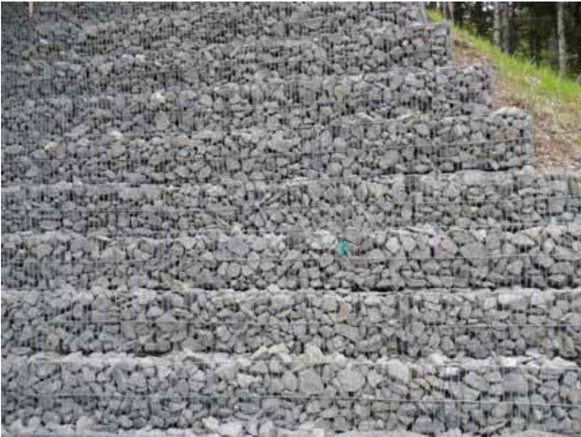
Figure 2-11. Wire gabion retaining wall structure.
