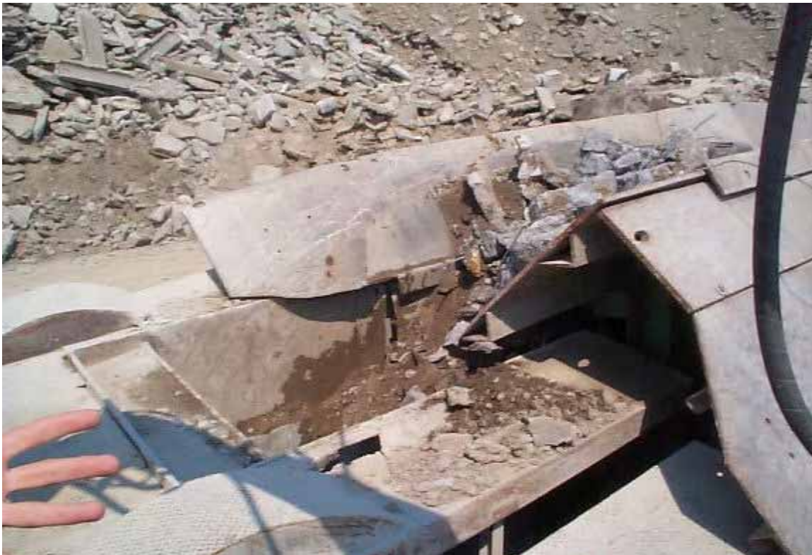
Figure 2-4. Primary jaw crusher for reduction of concrete size after (USDOT 2004).
