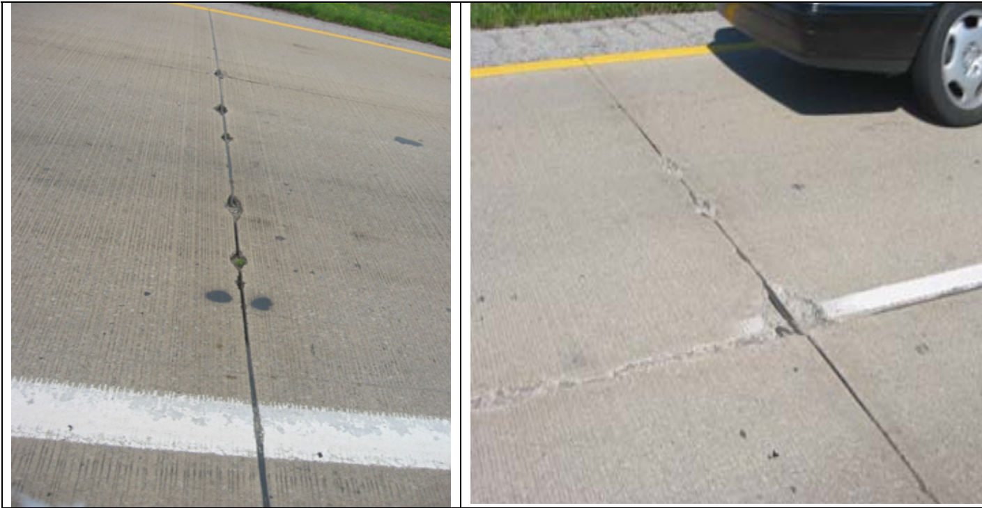
Figure 4.8 Joint spalling for test sections SHRP 260221 (a) and 260223 (b).
