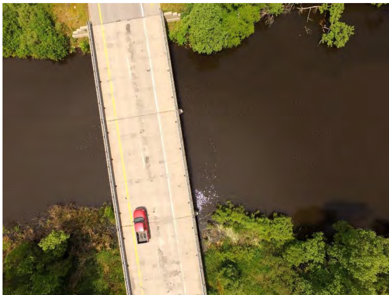
Figure 42: Example image from the Phantom 3A of the US-31 / White River bridge, taken while flying over water near the bridge.
