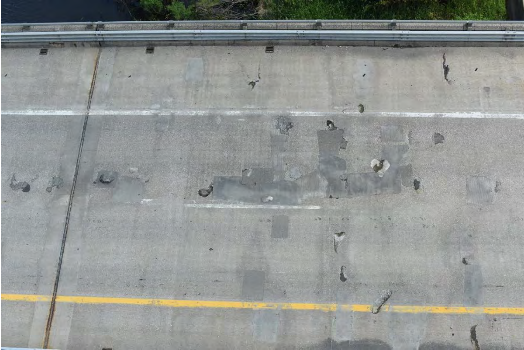
Figure 27: Bridge deck photo collected with Nikon D810 from the Bergen Hexacopter, used to create a detailed orthophoto and DEM of the bridge surface.
