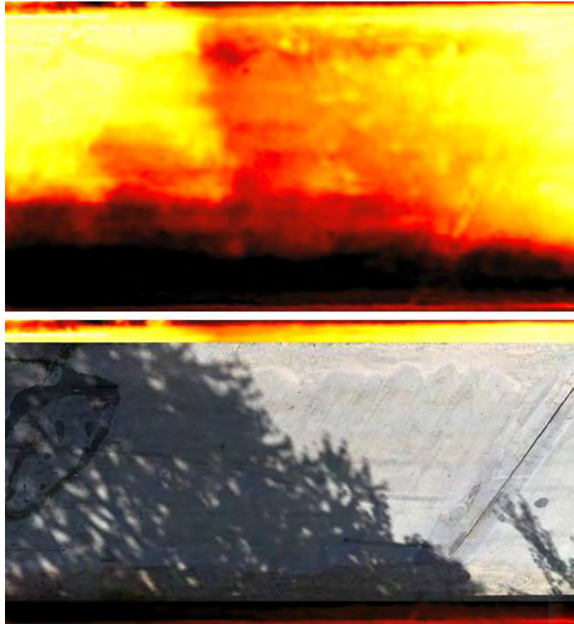
Figure 75: Comparison between the thermal (upper panel) and visible (lower panels) images at the Gordonville road test site. The presence of tree shadows, easily recognizable in the visible imagery (lower panel) mask the presence of potential thermal signatures related to delaminations (in the upper panel).
