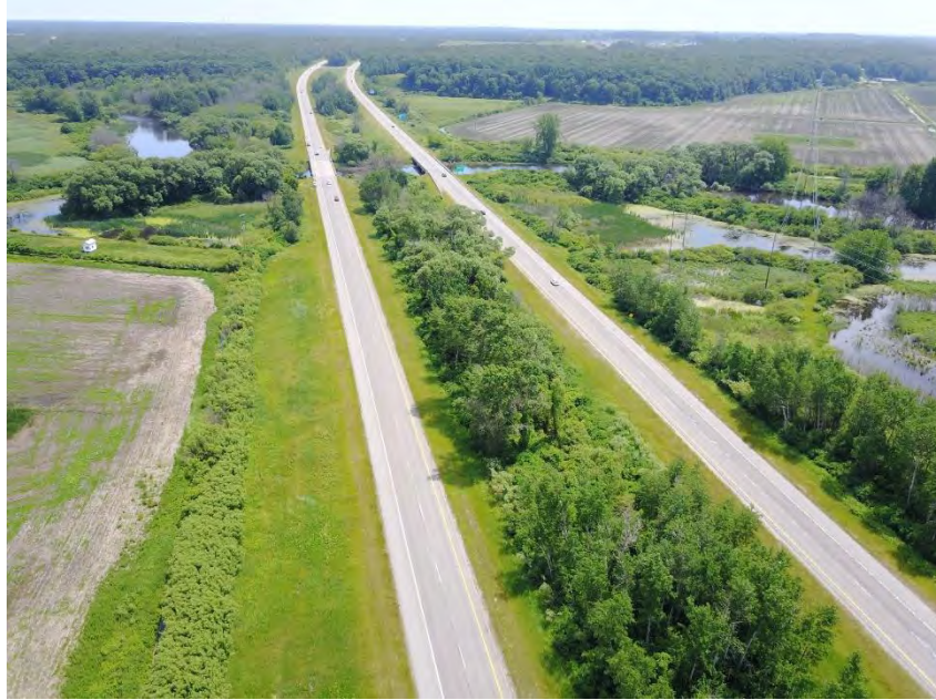
Figure 23: The main corridor area captured through use of US31 / White River site, as imaged by the Mavic Pro quadcopter. The left grassy area was used for UAV deployment, and the assessed bridge is visible over the White River in the background.
