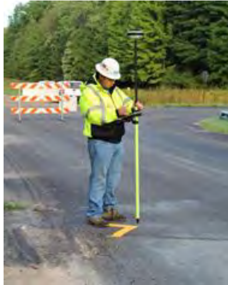
Figure 58: SSI team member A.Semenchuk collecting high accuracy GPS points.
