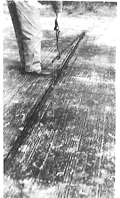
Pulling Tee Irons Prior to Removing Collapsible Joint Forms.
