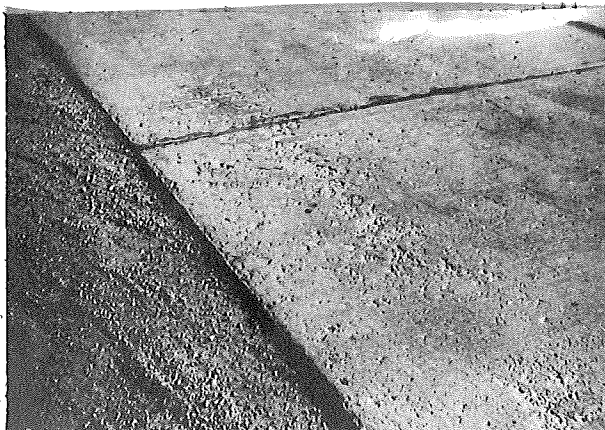
Typical Edge Scaling Stations 51+00 to 54+00 and 66+00 to 68+00
