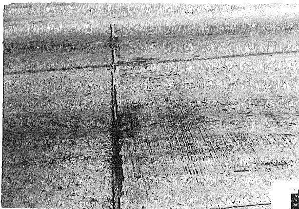
View of Expansion Joint with Wood Filler at Station 72+21
