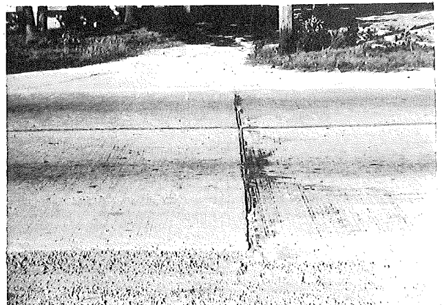
View of Expansion Joint with Wood Filler at Station 73+10
