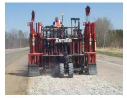
Pavement demolition equipment such as a multihead pavement breaker is used to break concrete into manageable fragments. Front-end loaders then haul these fragments to a crushing plant for processing into CCA.
