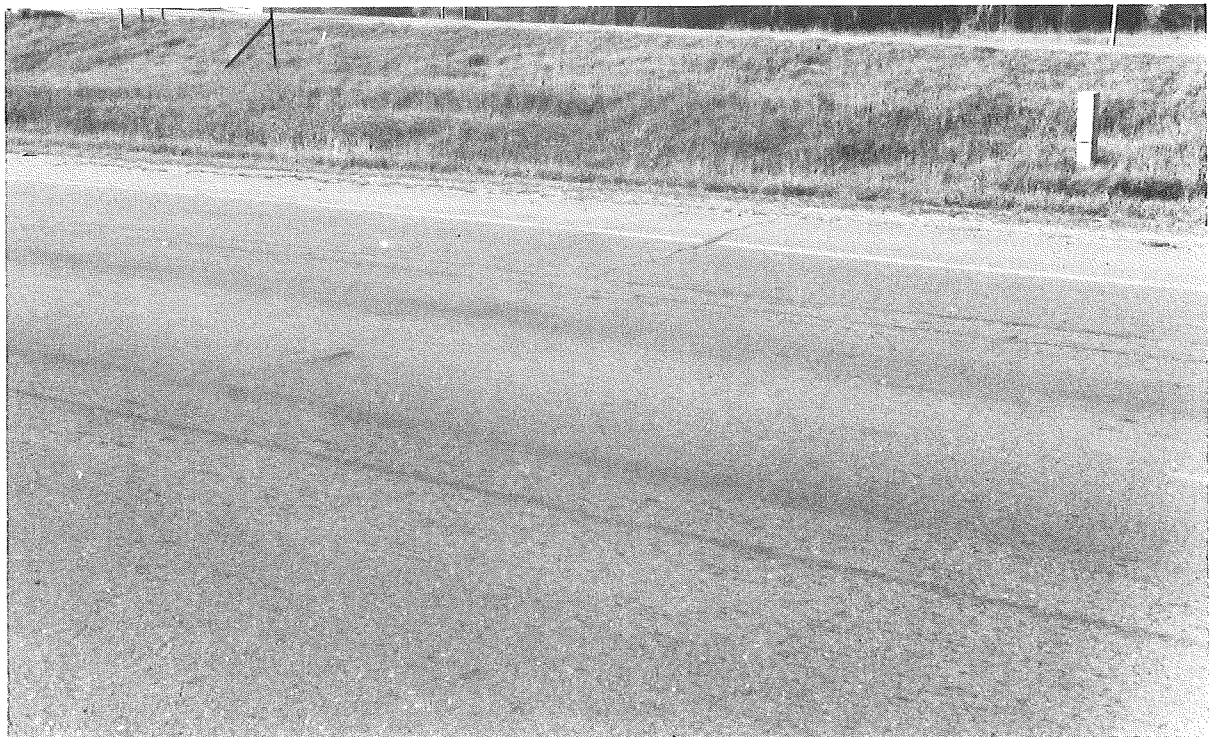
Figure 2. Condition of comparative sections at the time of final inspection, Fall 1983.
