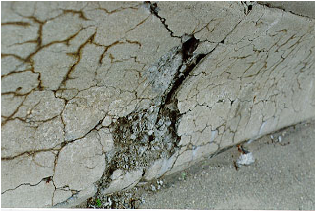
Figures 10A and 10B: Typical deterioration caused by freeze thaw attack.
