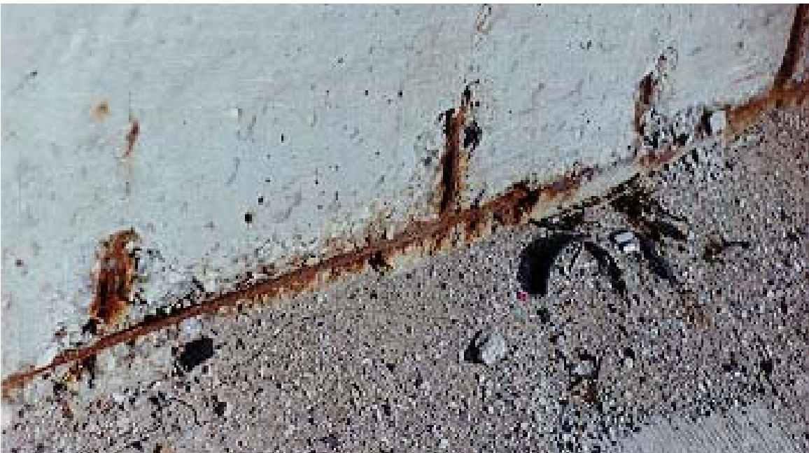
Figures 21A and 21B: Examples of corrosion of black reinforcing steel due to insufficient concrete cover.
