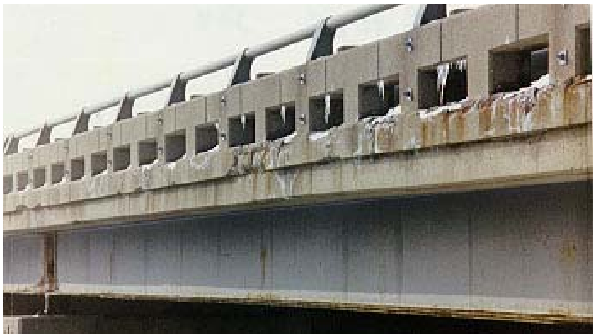
Figure 13A and 13B: Example of open parapet concrete railing retrofitted with beam guardrail.
