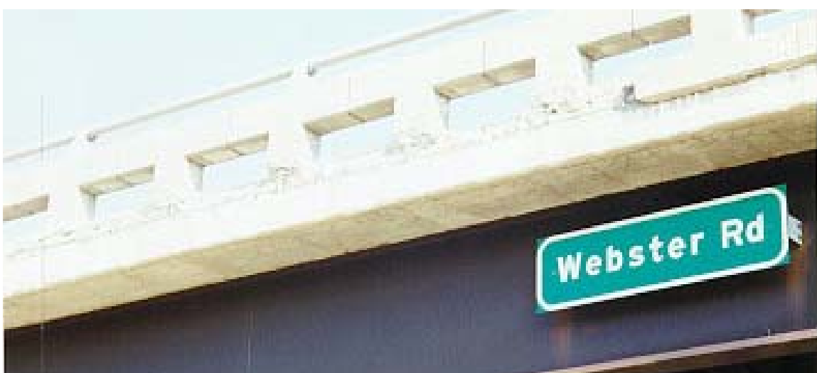
Figure 2A and 2B: Concrete railing typical of the standard R-11 or R-12 adopted in 1961.
