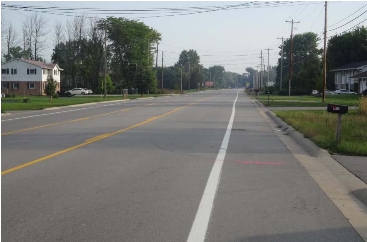
Figure 4.6: General Site Overview, M-84 in Bay City, Michigan
