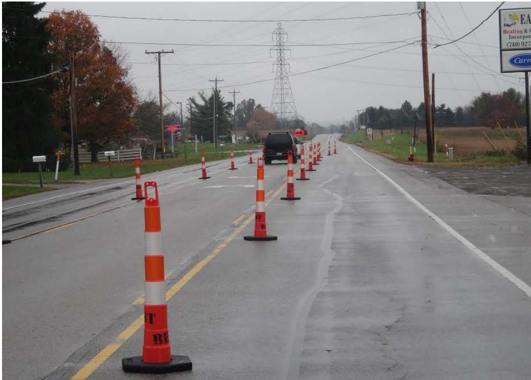
Figure 4.10: General Site Overview SR 310
