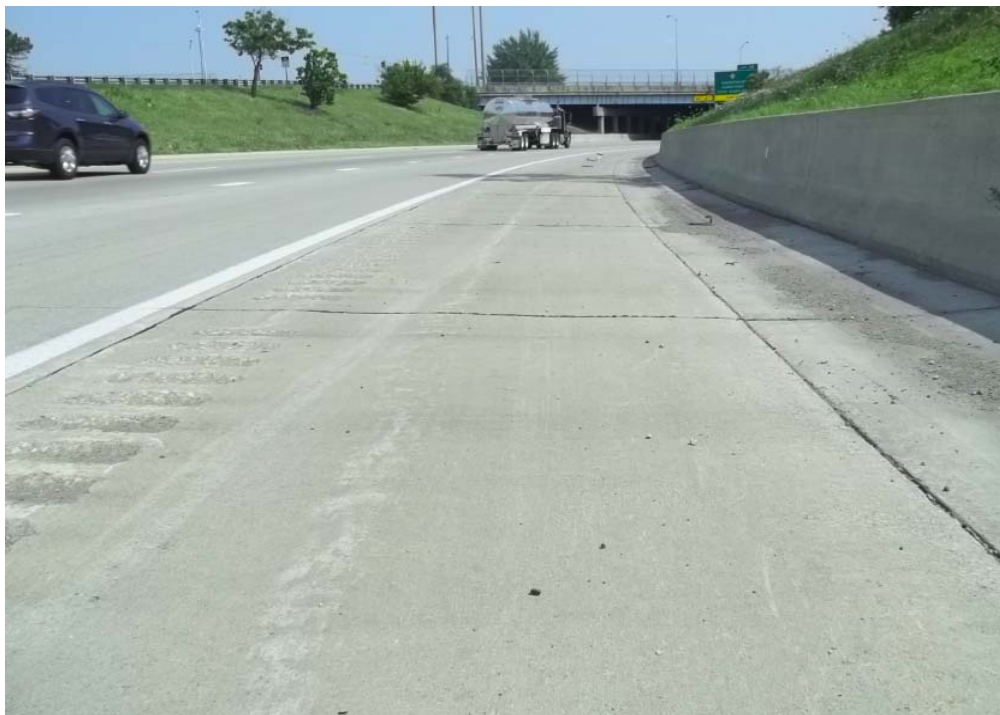
Figure 4.3: General Site Overview of I-75/I-96 Site
