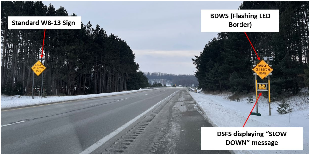
Figure 13. Example of Active BDWS and DSFS at SB US-131 Cadillac Site
