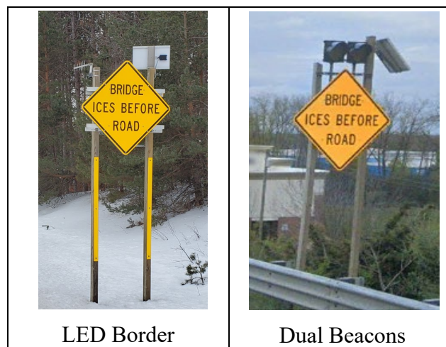
Figure 68. Static Sign with LED Border and Dual Beacons
