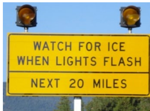
Figure 5. Ice Warning Signs with Flashing Beacons Used in Oregon (Veneziano & Ye, 2011)
