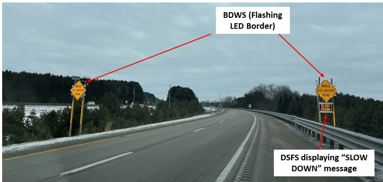
Figure 11. Example of Active BDWS and DSFS at NB US-131 Cadillac Site
