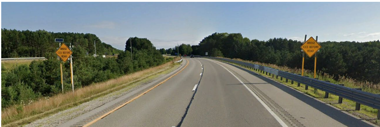
Figure 61. BDWS Signage on NB US-131 at E. 50 Road
