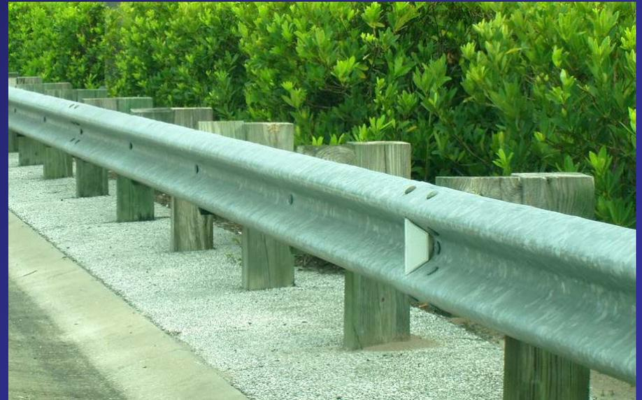
Delineators should be used with guardrails and other barriers
