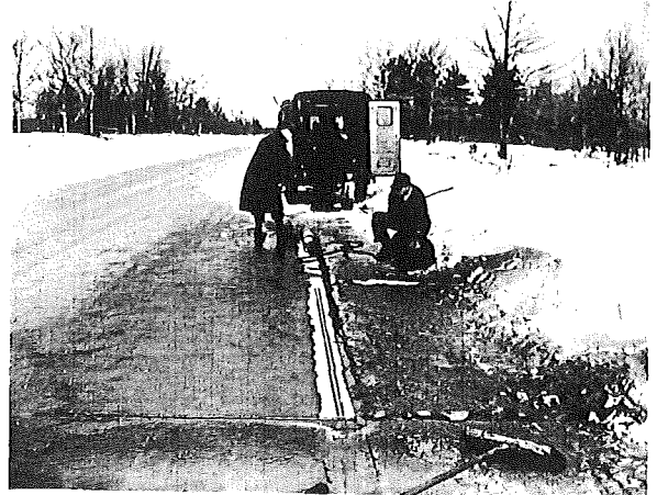
B. DRYING PAVEMENT SURFACE PRIOR TO INSTALLING DYKE STRIPS
