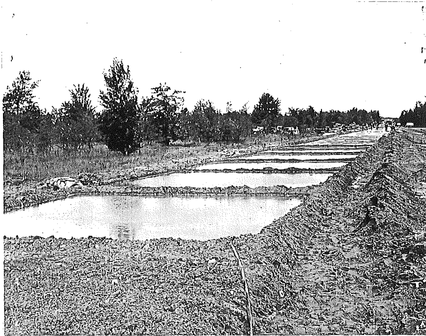
A. General View of Curing Section
