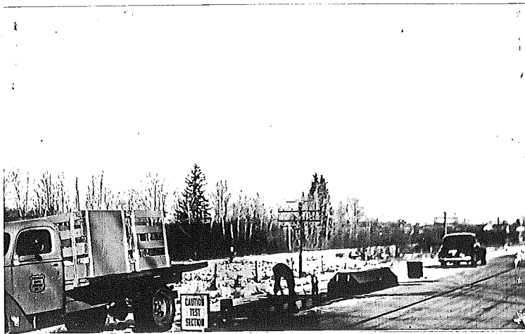
B. General View Showing Metal Hood used in "Method B", Baraga Project US-41
