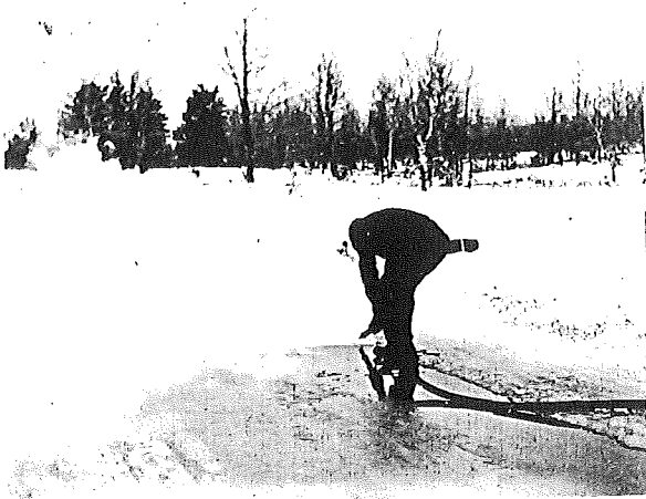
A. IN 1940-1941- STEAM WAS USED TO REMOVE ICE FROM PAVEMENT PRIOR TO INSTALLING PANEL STRIPS
