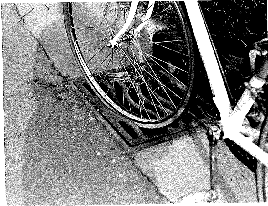
Figure 1. Racing bicycle tire penetrating opening in sinusoidal type grating.
