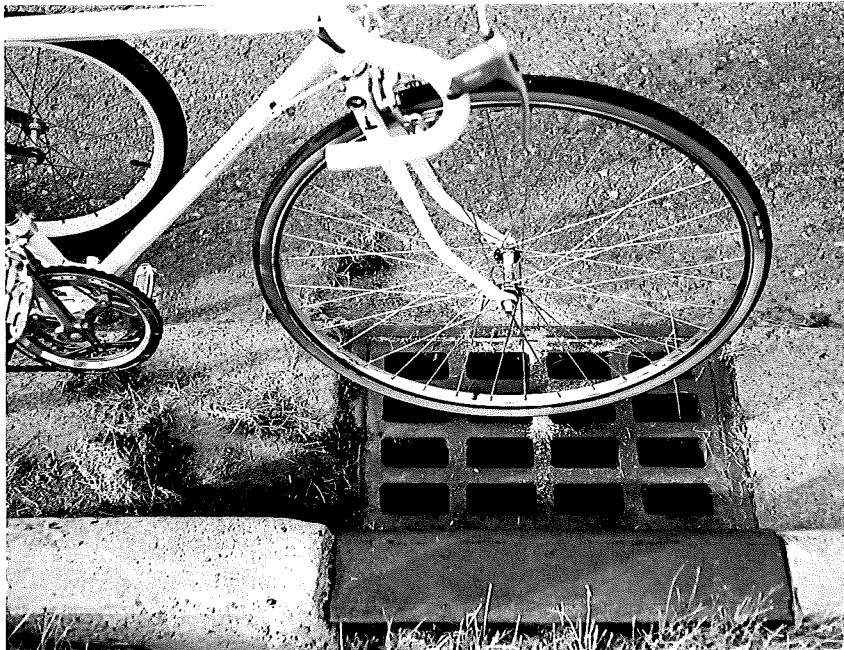
Figure 2. Same bicycle tire on rectangular grating.
