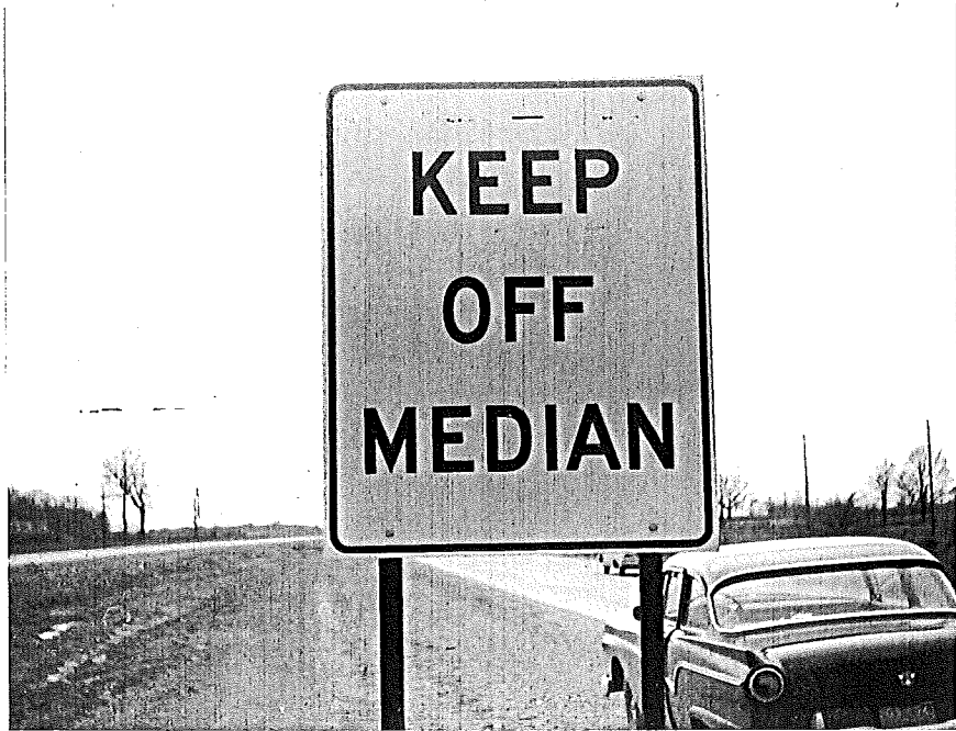
Figure 3. Black paint and white reflectorized background on plywood.
