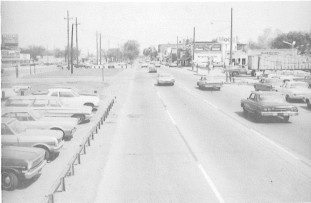
FIGURE #3 M-85 (Fort St.) @ Oak St. looking north before the construction improvement.
