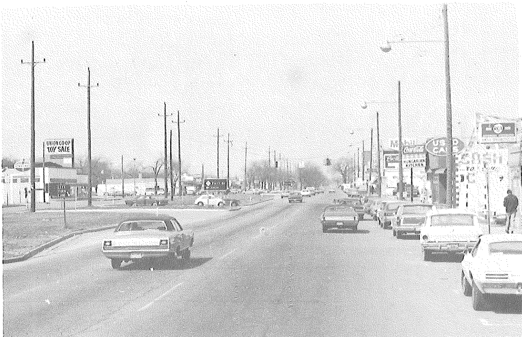
FIGURE #4 M-85 @ Oak Street looking north after the improvements.
