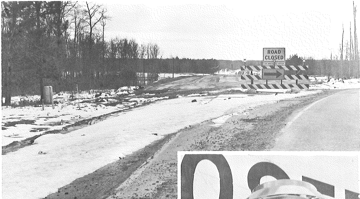
▲ Figure 1. Propane lights on M 18 road closure. Supply tanks at left center.
