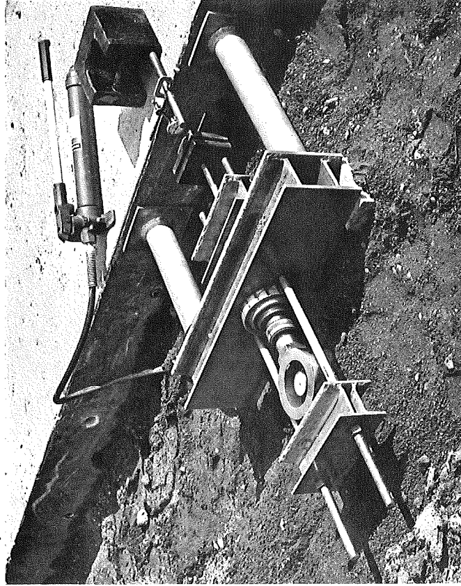
Figure 2. 20,000-lb capacity test frame used to apply load to the anchors.
