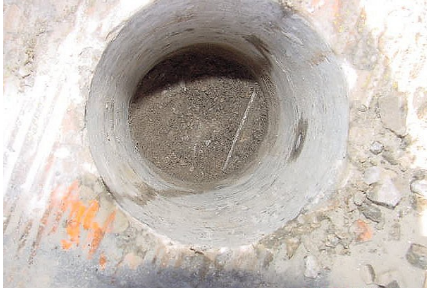
Figure 3.4a Core hole showing support angle in flange up position.
