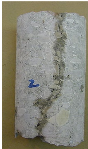
Figure 3.4b Core through full depth longitudinal crack.
