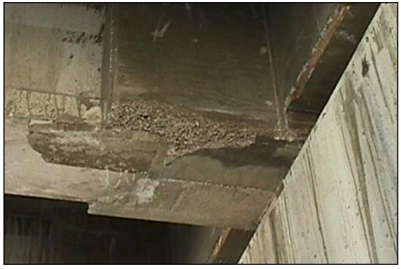
**Figure 6 -** Exposed aggregate.
