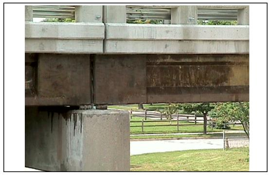
**Figure 8 -** Appearance of concrete penetrating epoxy sealer.
