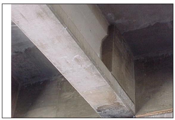
**Figure 5 -** Bevel only on horizontal lower portion near bottom flange.
