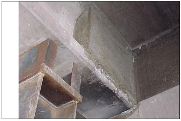
Figure 4 - Bevel only along vertical exterior corner of web.
