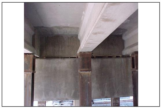
**Figure 7 -** End diaphragm too close to top of pier.
