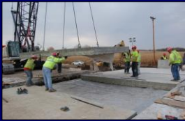
Precast Approach Slabs
