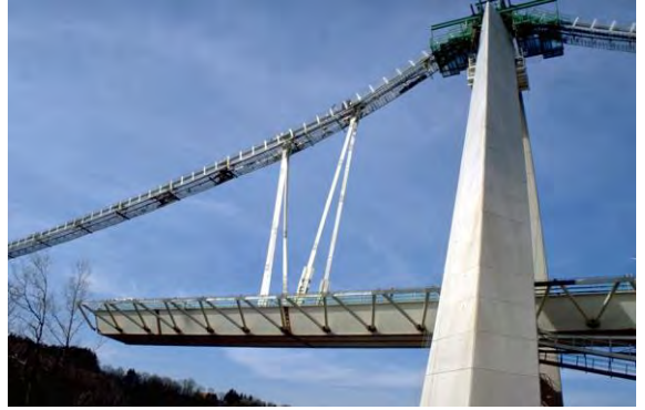
Temporary Hangers 2– Stage
