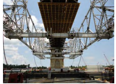
Straddle Widening Trusses
