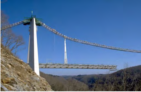
Temporary Hanger – Stage 1
