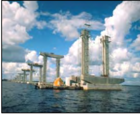
Prefabricated Piers (columns/caps)
