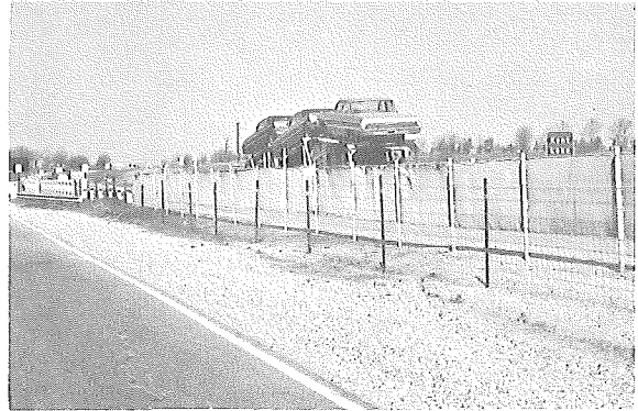
Anti-Glare Screen viewed at 15° angle from Service Road.
