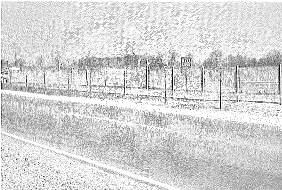
Anti-Glare Screen viewed at 25° angle from Service Road, westbound.
