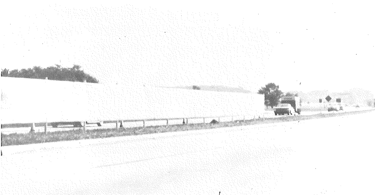
Close up view of Anti-Glare Screen in Median of I-96 at Kent Lake Road.
