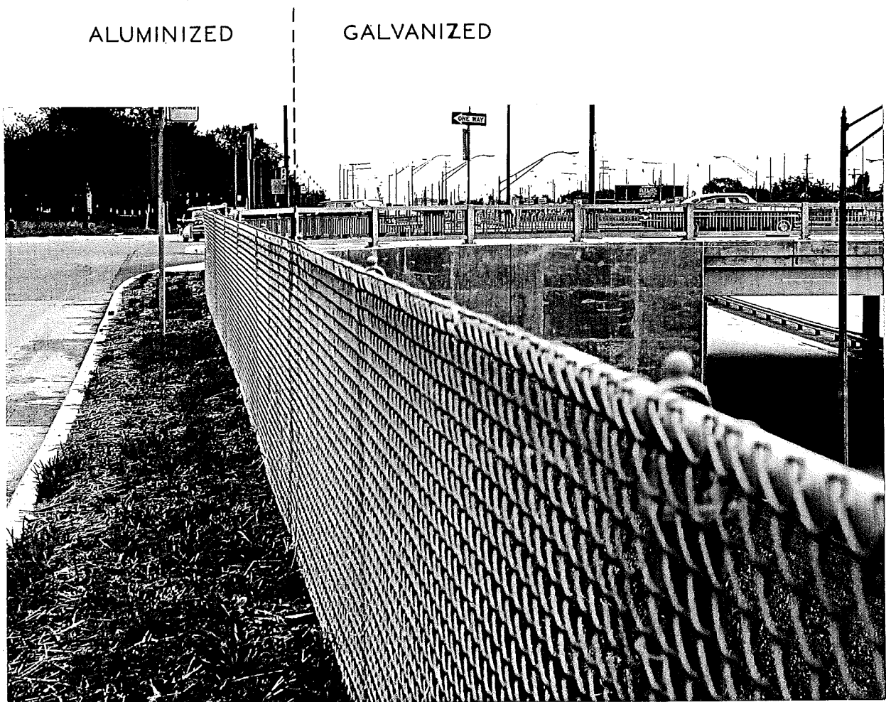
Figure 1. Field installation at Southfield Freeway and Plymouth Rd six months after installation. Aluminum coated fencing in background and zinc-coated in foreground.
