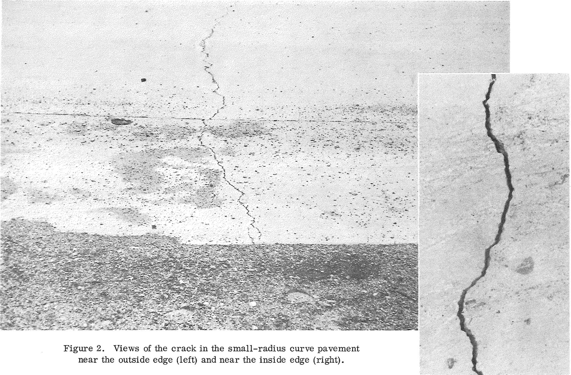
Figure 2. Views of the crack in the small-radius curve pavement near the outside edge (left) and near the inside edge (right).
