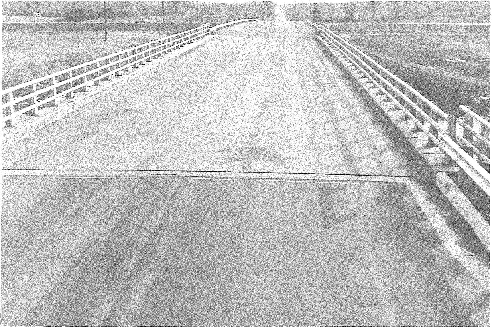
Figure 1. View looking south over Crietz Rd Bridge, December 1969.
