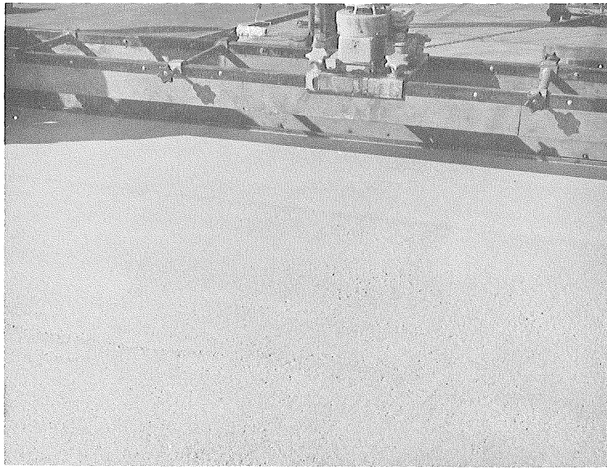
Rough texture of fresh epoxy mortar immediately behind the screed machine.
