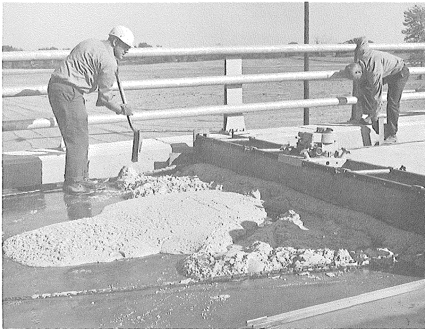
Distributing the epoxy mortar ahead of the screed.
