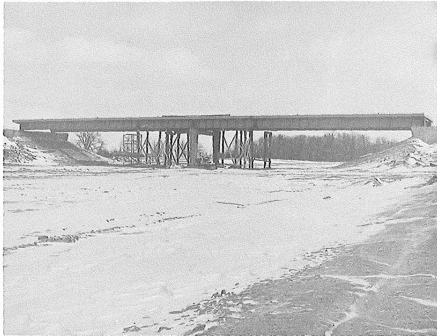
General view of the structure with all nine deck sections field bolted.
