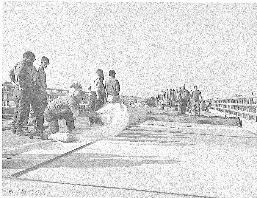
Broadcasting silica sand on top of the fresh mortar for maximum skid resistance.
