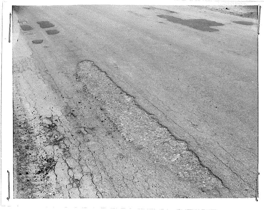
Figure 9. Break in seal coat at Station 45+00 showing condition of stabilized base. The light spots are pieces of mineral filler not thoroughly mixed with the soil. The bituminous binder, not evident in picture, also was not intimately mixed with the sand. At this point the stabilized base showed a small amount of cohesiveness, but was also comparatively soft.
