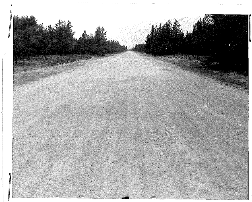
Figure 14. View from the east end of the project looking west. Surface is in excellent condition.
