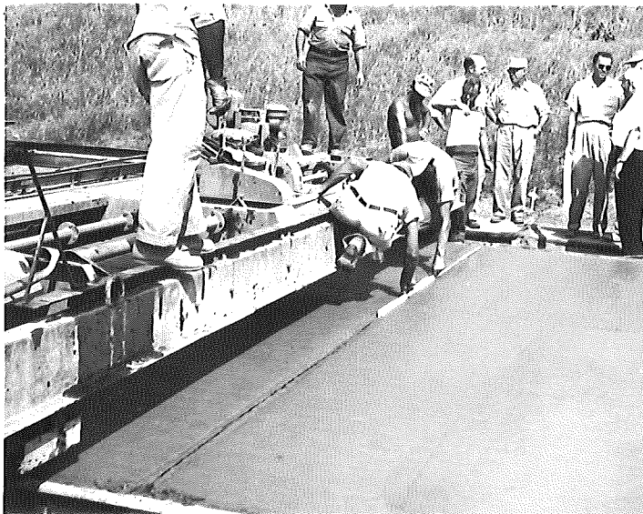
▲ FIGURE 3. INSERTING STYROFOAM FILLER.
