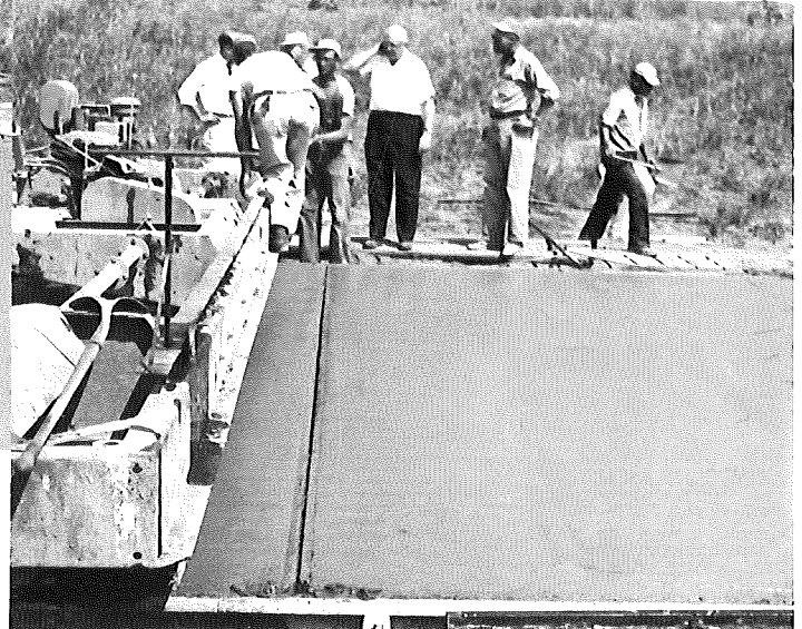
▲ FIGURE 2. GROOVE READY TO RECEIVE FILLER MATERIAL.
