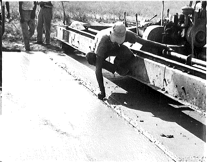
▲ FIGURE 9. COMPLETED INSTALLATION OF CORRUGATED PAPER BOARD.
