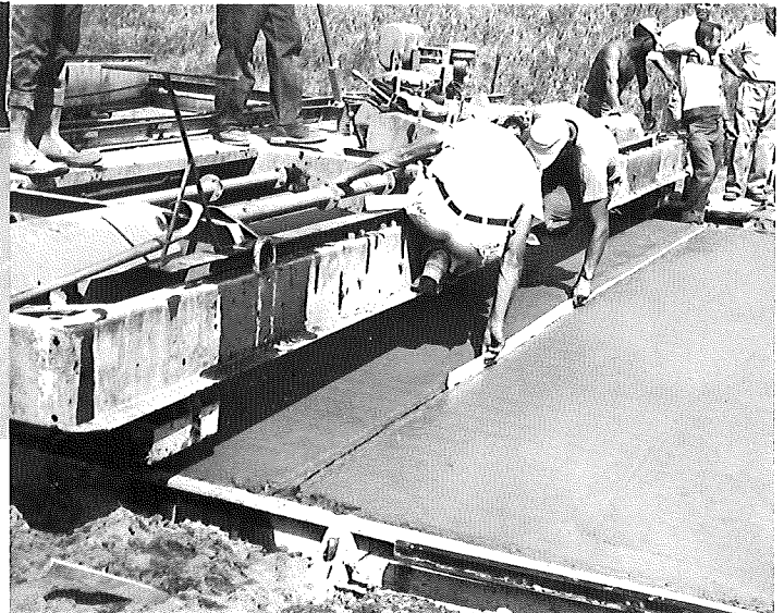
▲ FIGURE 4. INSERTING STYROFOAM FILLER.
