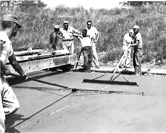
▲ FIGURE 6. FLOATING AND STRAIGHT-EDGING CONCRETE AT STYROFOAM JOINT.
