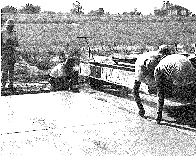
▲ FIGURE 8. INSERTING CORRUGATED PAPER BOARD.
