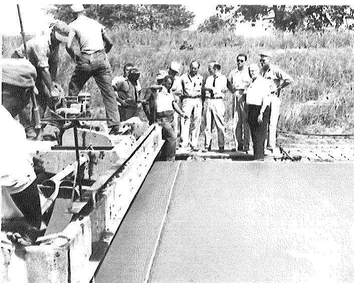
▲ FIGURE 4. INSERTING STYROFOAM FILLER.
