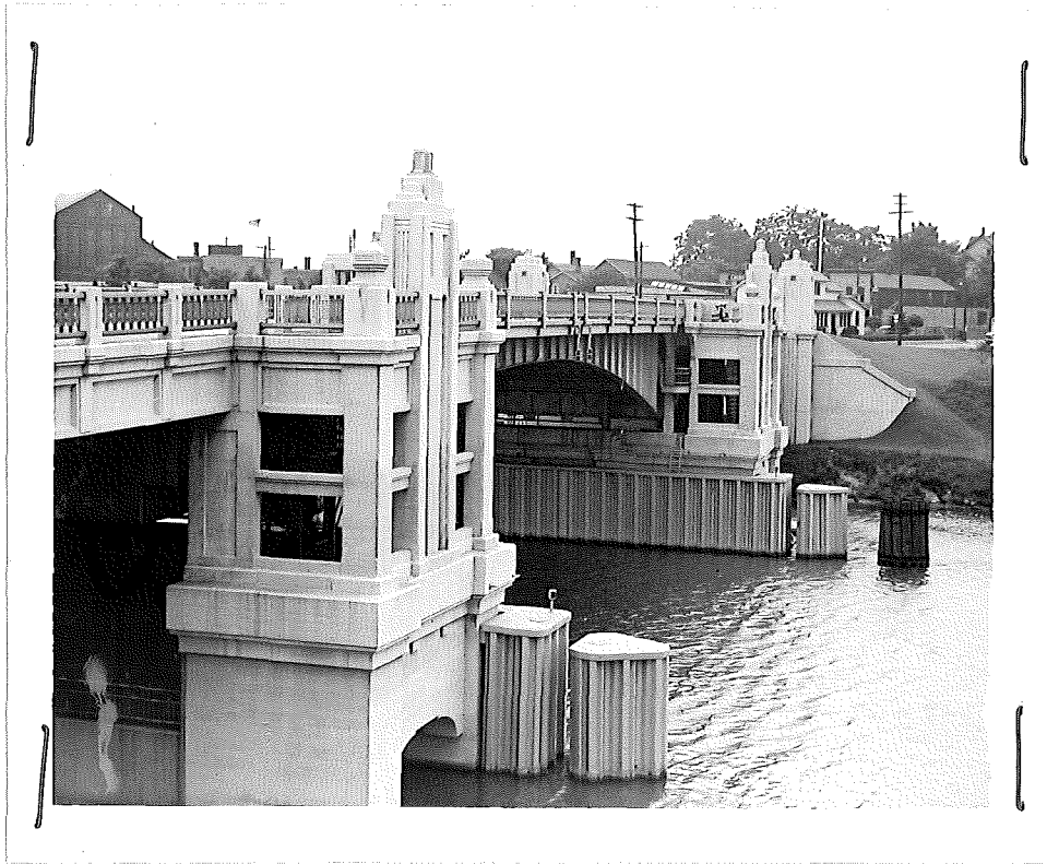
Figure 3. General view of bridge at Manistee. Painted in 1945 with Peerless portland cement paint.
