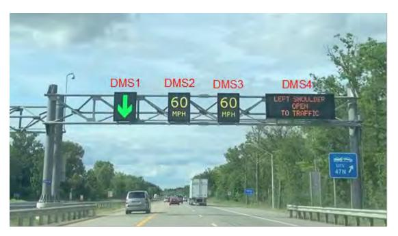
Figure 3-7 An example of gantry messages on the US-23 Flex route (NB MM46.8)
