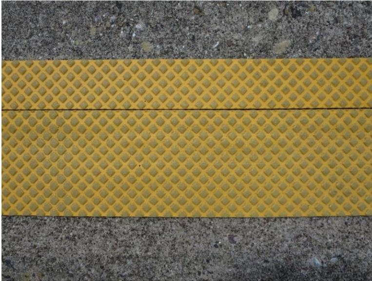
**Figure 7. Example 4- and 2-inch Sections of the Preformed Tape Pavement Marking**
