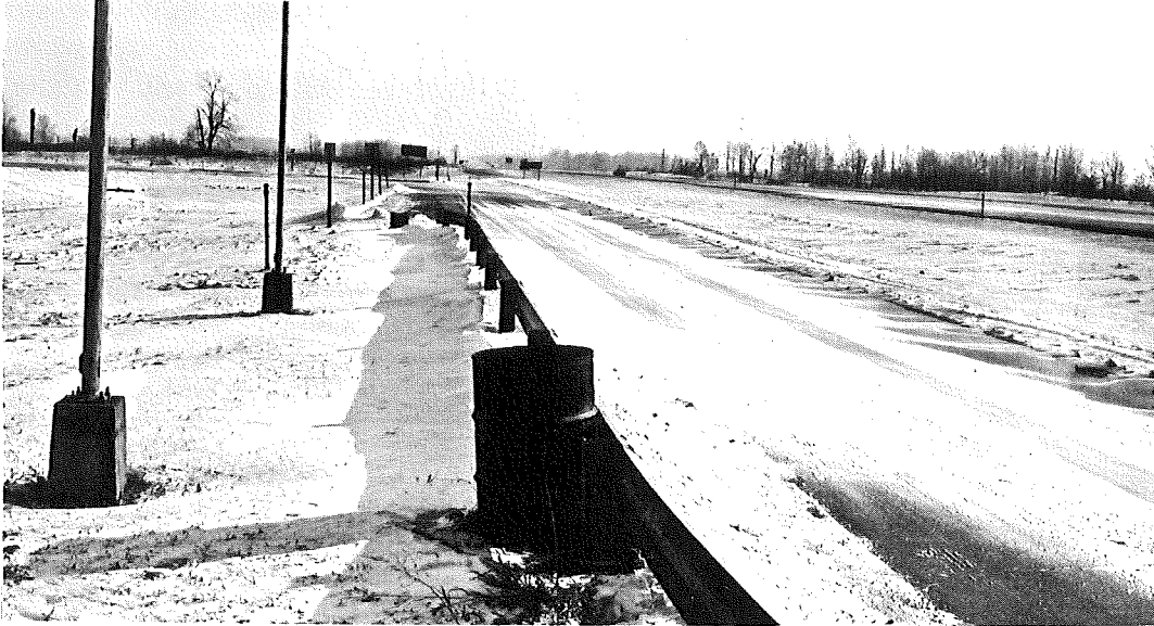
Figure 6. Build-up of blowing snow on chemically treated test section.
