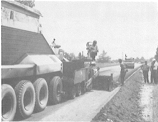
Photo 12. Paving operation.
