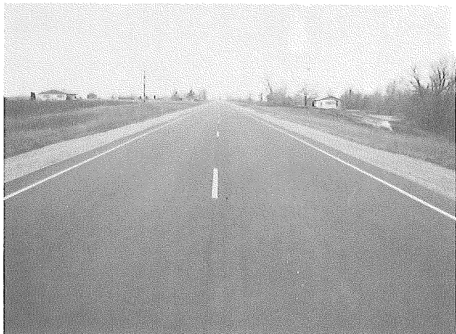
Photo 14. M 57 After. Two 12 ft lanes with 3 ft paved shoulders.
