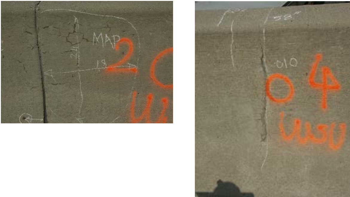
Figure A-50. Core specimen locations for S06-82022, H1 (left) and H2 (right).
