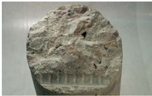
Figure A-3. Imprint of rebar in core A2.
