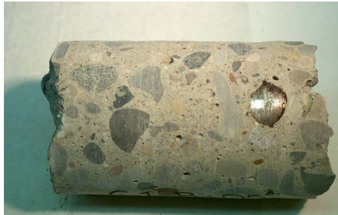
Figure A-29. Core E2 (bottom part), corrosion of reinforcing steel.
