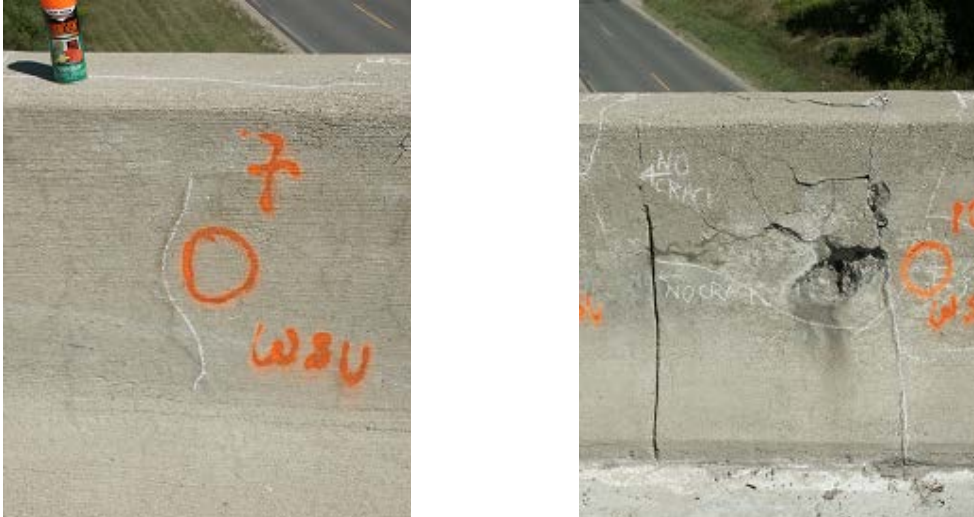
Figure A-43. Core specimen locations for S01-44044, G1 (left) and G2 (right).
