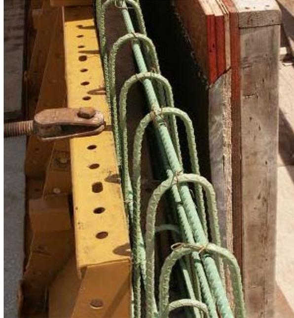
**Photo 5-2. Formwork of barriers of bridge S05–82191**
