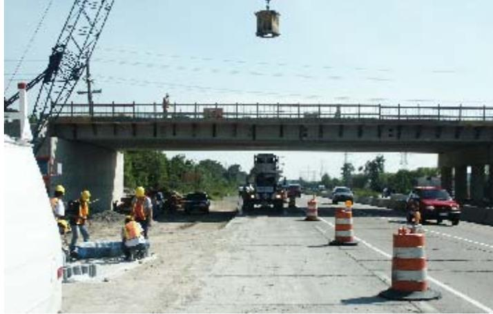
**Photo 5-5. Concrete placement with bucket (S05-82191)**
