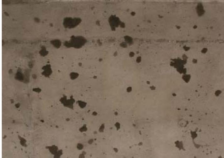
**Photo 5-12. Repaired surface voids of form-cast barrier surface (S05-82191)**
