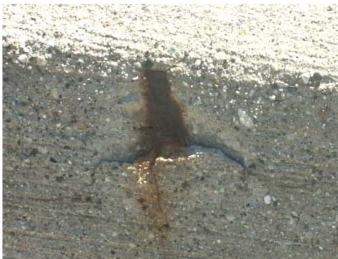
Signs of corrosion due to lack of concrete cover
