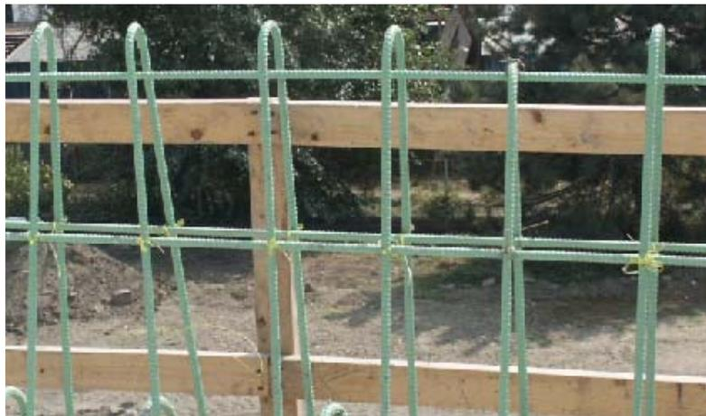
Photo 5-1. Reinforcement ties missing at some rebar intersections (bridge S06-82194)
