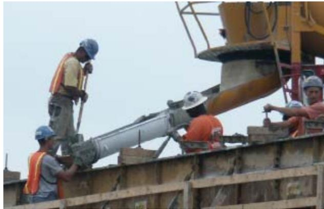
**Photo 5-6. Concrete placement directly from mix-truck (S20-50111)**
