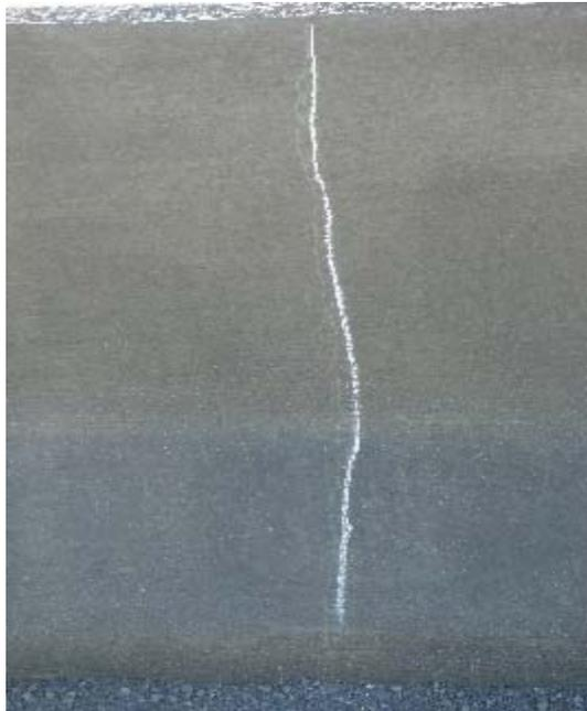
**Photo 5-21. Full-length vertical crack on the barrier observed 48 hours after slipforming (S06-82194)**
