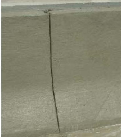
**Photo 5-17. Hand finish joint of a slipformed barrier (S06-82194)**
