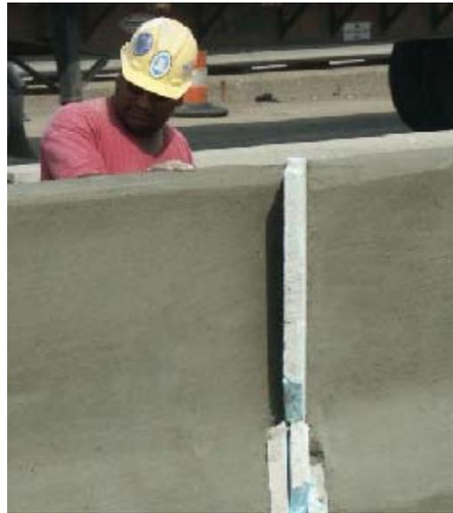
**Photo 5-16. Portions of plastic concrete near the construction joint of slipformed barrier broke away and later hand repaired (S06-82194)**
