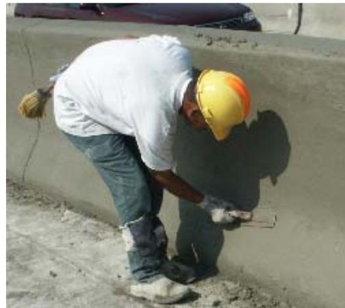
**Photo 5-11. Surface finishing of slipformed barriers (S06-82194)**
