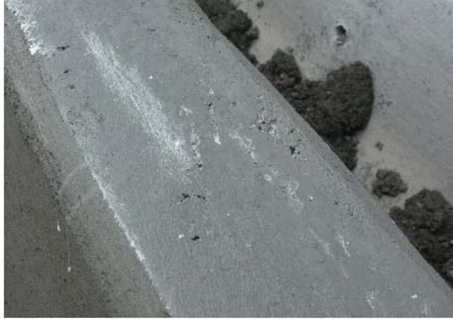
**Photo 5-15. Visible surface defects after extrusion in slipformed barriers (S06-82194)**
