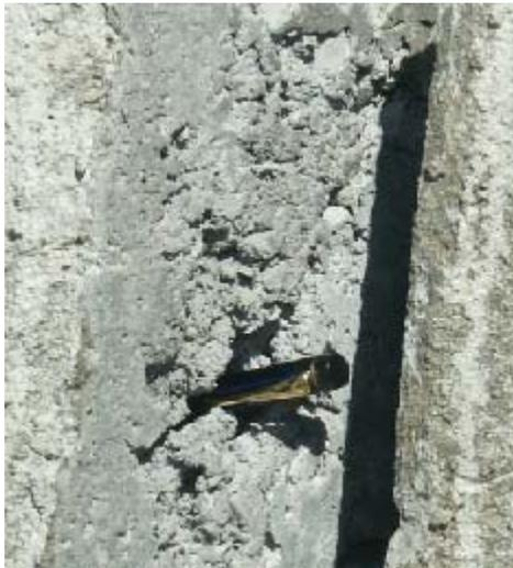
**Photo 5-18. Honeycombing and large voids were visible at the joint of slipformed barrier (S06-82194)**
