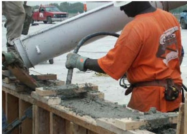
**Photo 5-7. Concrete consolidation using vibrator (S20-50111)**
