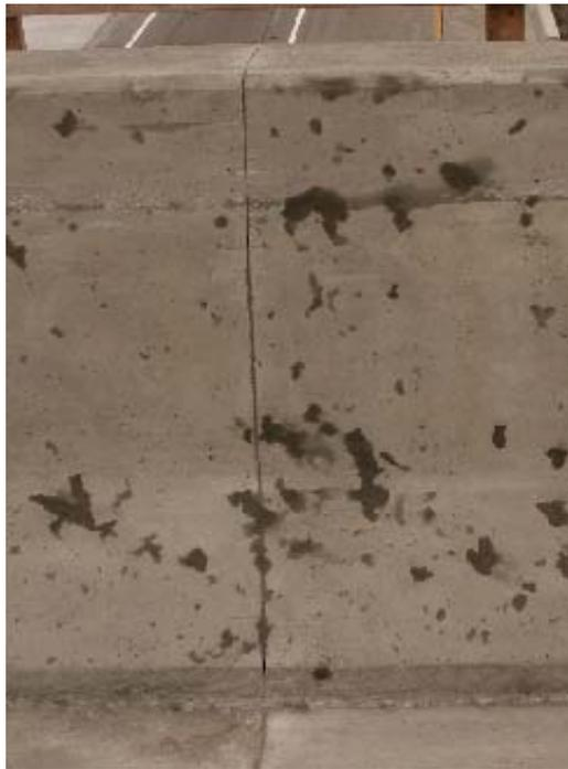
**Photo 5-13. Saw-cut joint of a form-cast barrier (S05-82191)**
