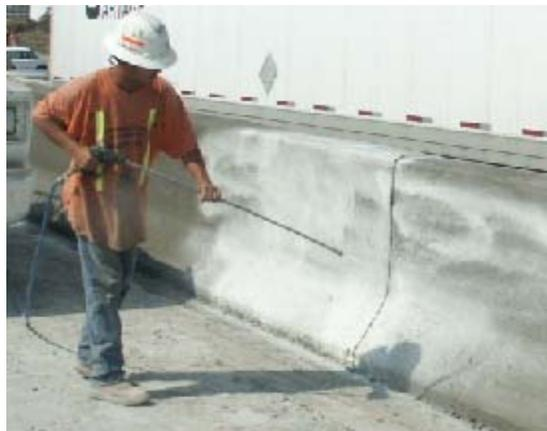
**Photo 5-19. Application of the one and only layer of curing compound on barrier surface (S06-82194)**
