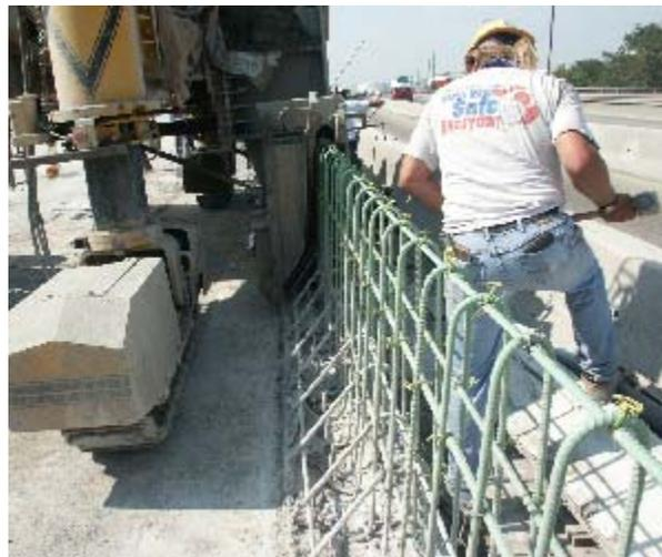
**Photo 5-10. Realigning rebar by hammering (S06-82194)**
