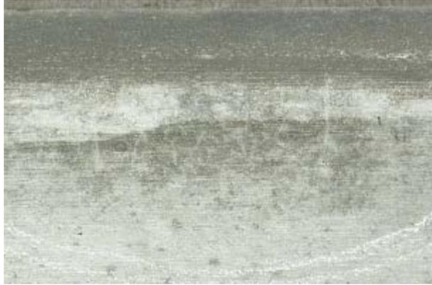
**Photo 5-20. Map cracking of barrier surface observed 48 hours after slipforming (S06-82194)**
