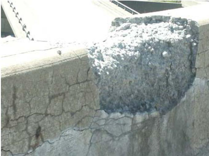
Severe section loss at or near the top of the barrier
