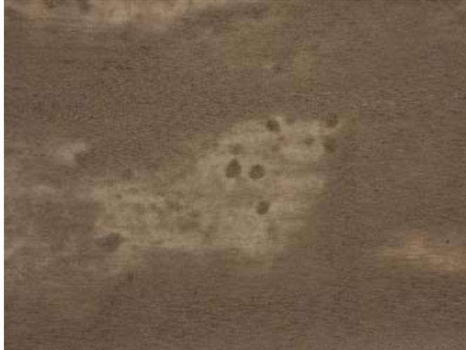
**Photo 5-14. Barrier surface without curing compound the day after concrete placement (S05-82191)**
