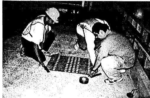
(b) Placing the UPV Template
