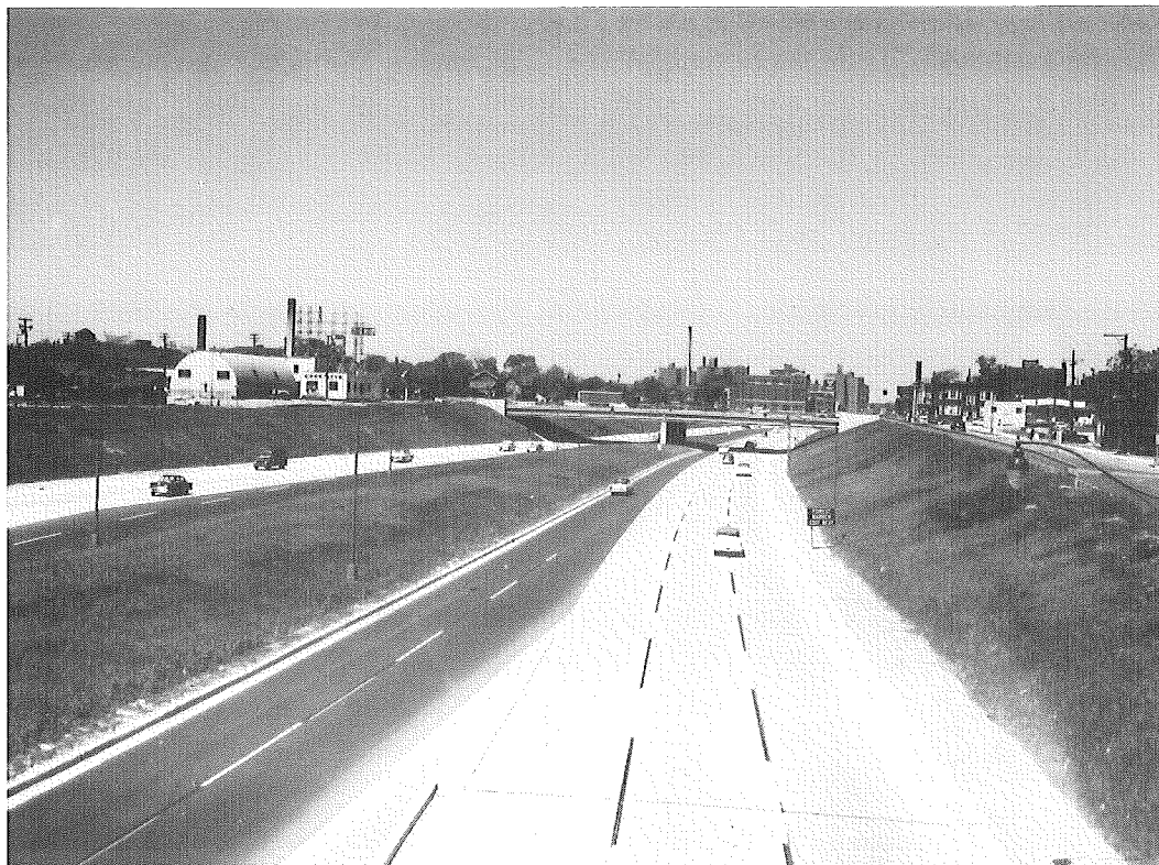
Figure 4. Six-lane expressway, showing black-white lane lines and the use of black pigmented concrete to channel traffic.
