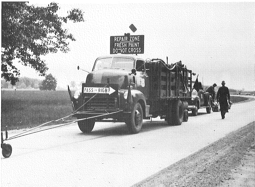
Figure 6. Front quarter view of striping equipment used by Michigan State Highway Department.
