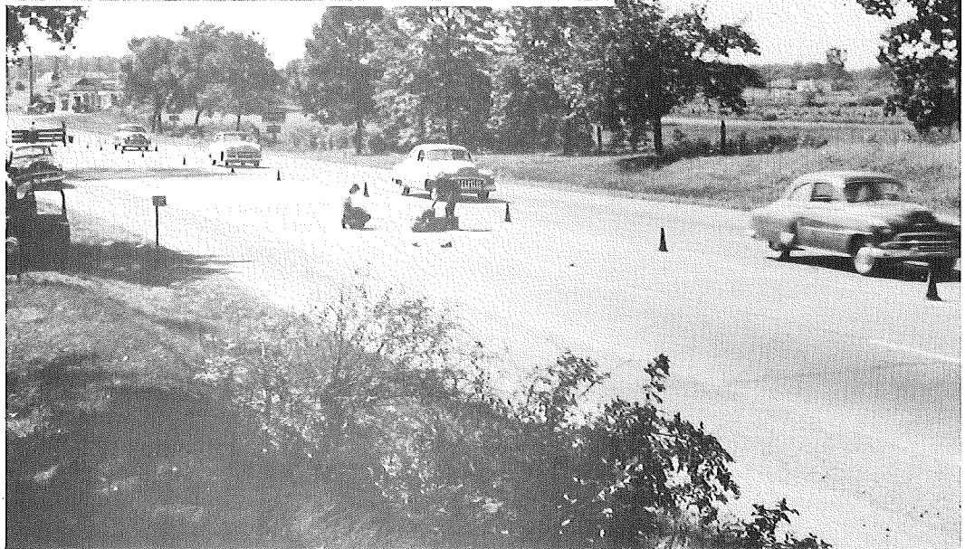
Figure 8. General view of paint test section.
