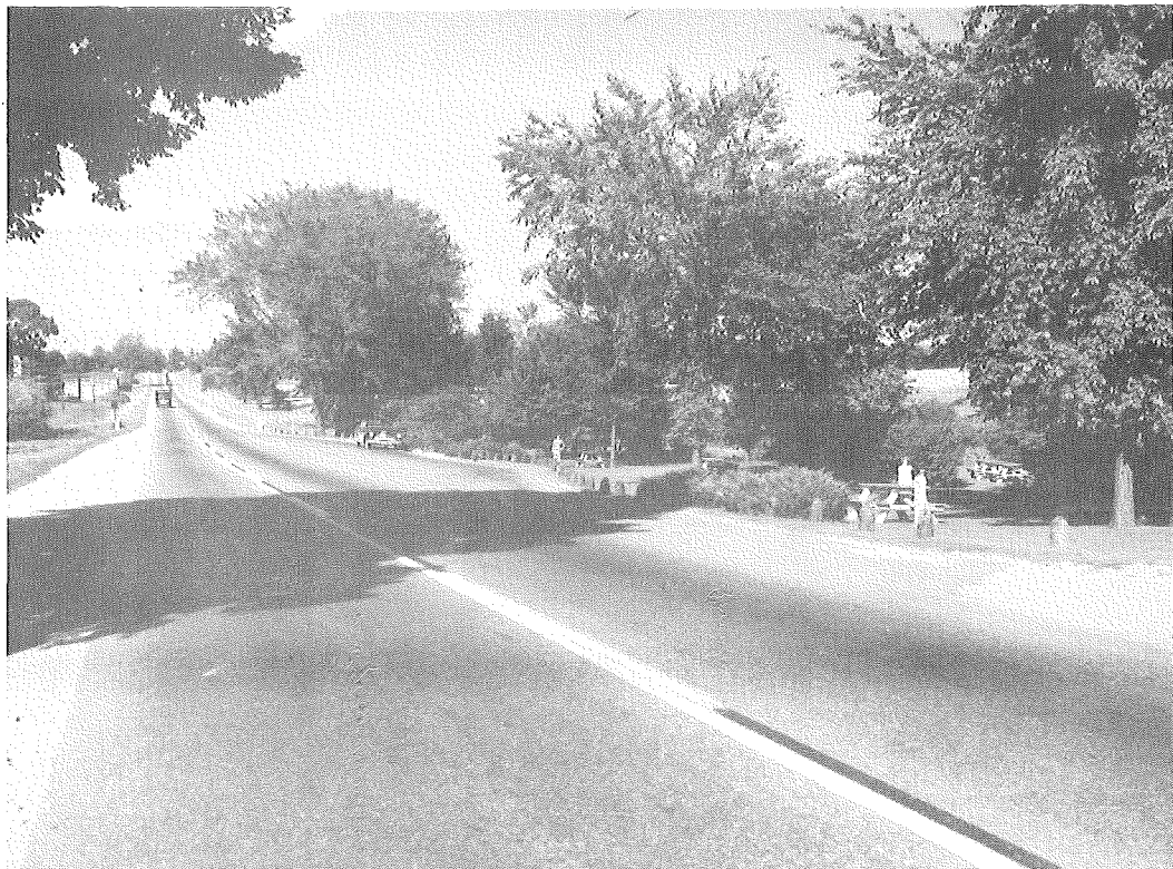
Figure 2. Two-lane bituminous concrete with black-white skip centerline (right) and solid yellow no-passing line (left).
