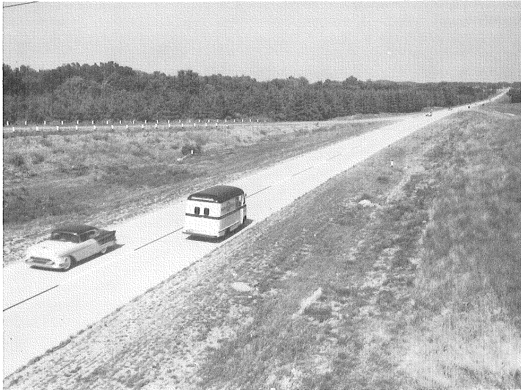
Figure 3. Two-lane concrete pavement with black-white centerline. The black segment is effective here.
