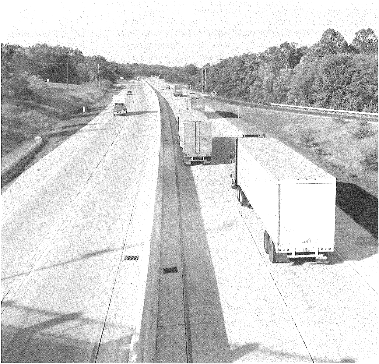
MDOT and the Transportation Commission are concerned with increasing numbers of truck accidents.
