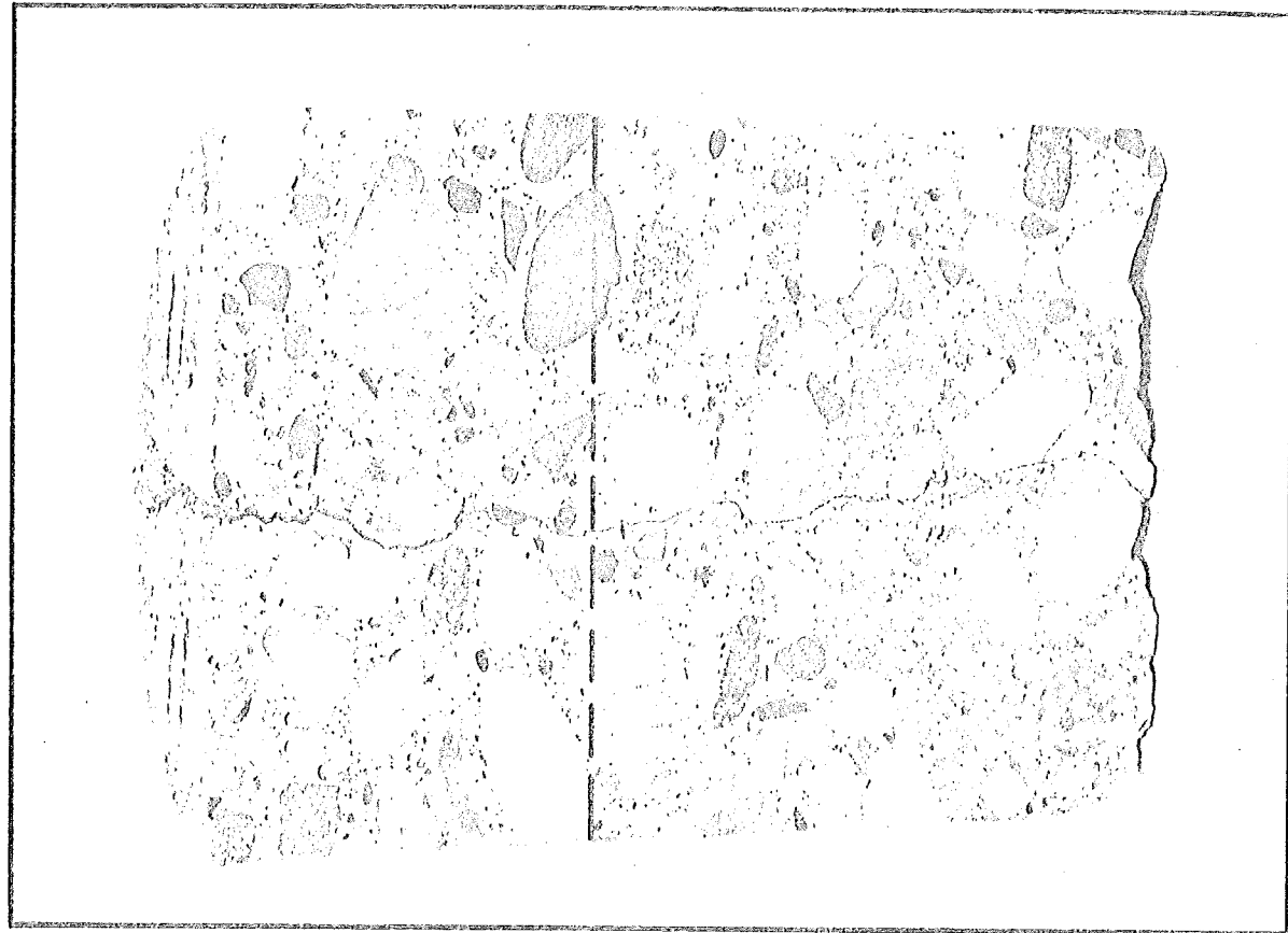
Figure 23. Typical appearance of crack widths in bar mat (left) and wire mesh (right) reinforced pavement after 10 years of service.
