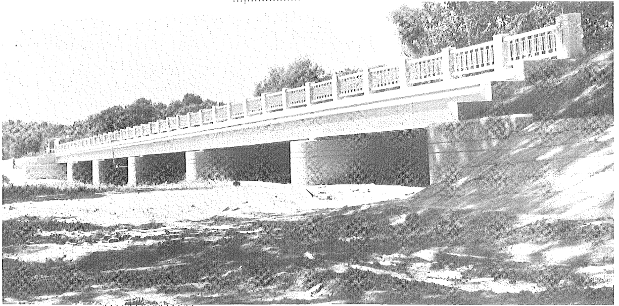
▲ FIGURE 2. GENERAL VIEW OF BRIDGE AT TIME OF TEST
