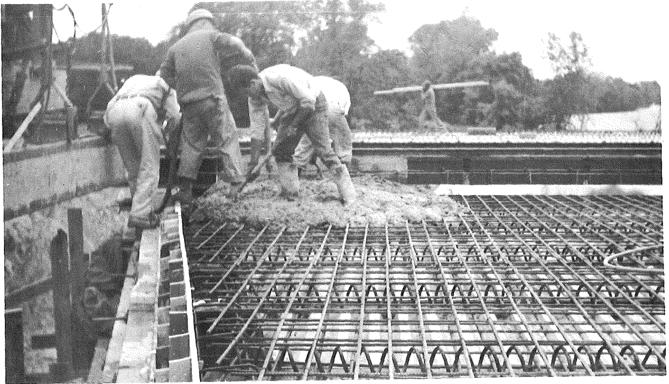
Figure 7. Placing concrete on Span 1.
