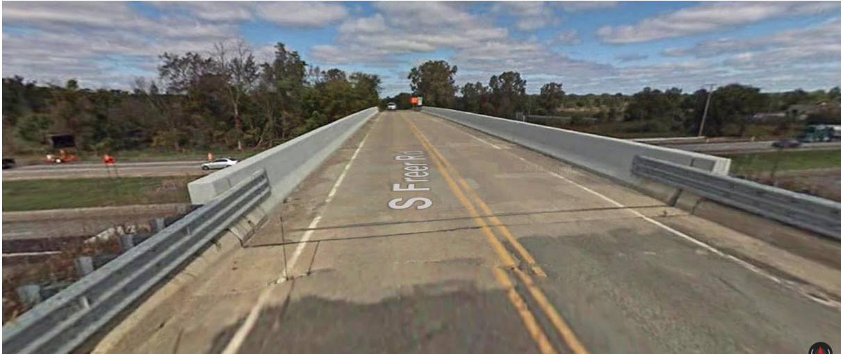
Figure 4-16: Bridge Deck of Freer Road Bridge.
