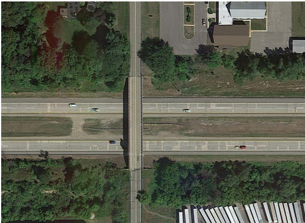
Figure 4-12: Maryland Ave. Bridge over I-196 Located in Kent County, Michigan
