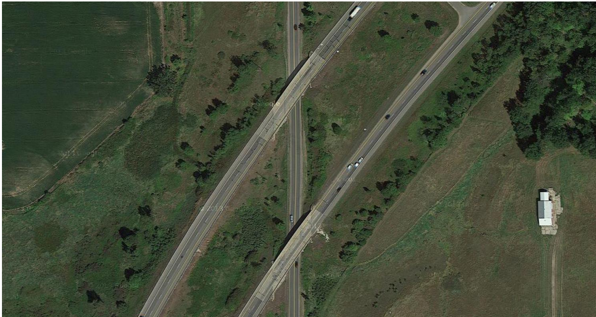
Figure 4-7: North and South Bound US-131 Bridges over White Creek Ave. near Cedar Springs, Michigan.
