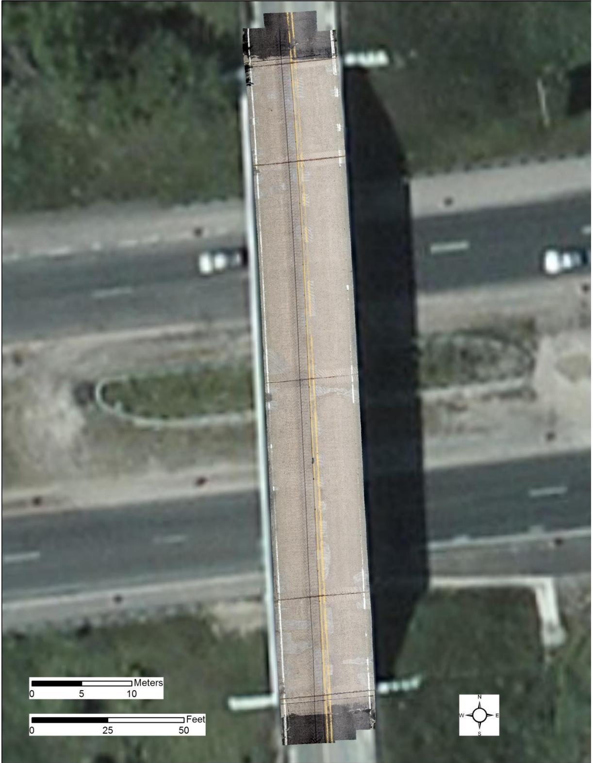
Figure 5-1: Orthoimage of Freer Rd Generated from Imagery Collected from the RED Epic.
