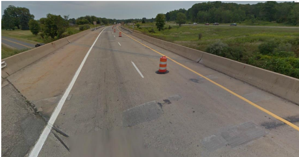
Figure 4-8: MDOT Structure No. 5002 SB US-131 Bridge Deck.
