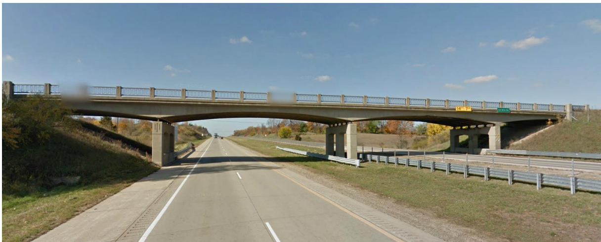
Figure 4-4: 24 Mile Road Bridge Selected as a Fall 2013 Deployment Site.
