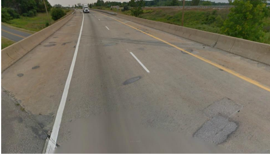
Figure 4-9: MDOT Structure No. 5003 NB US-131 Bridge Deck.
