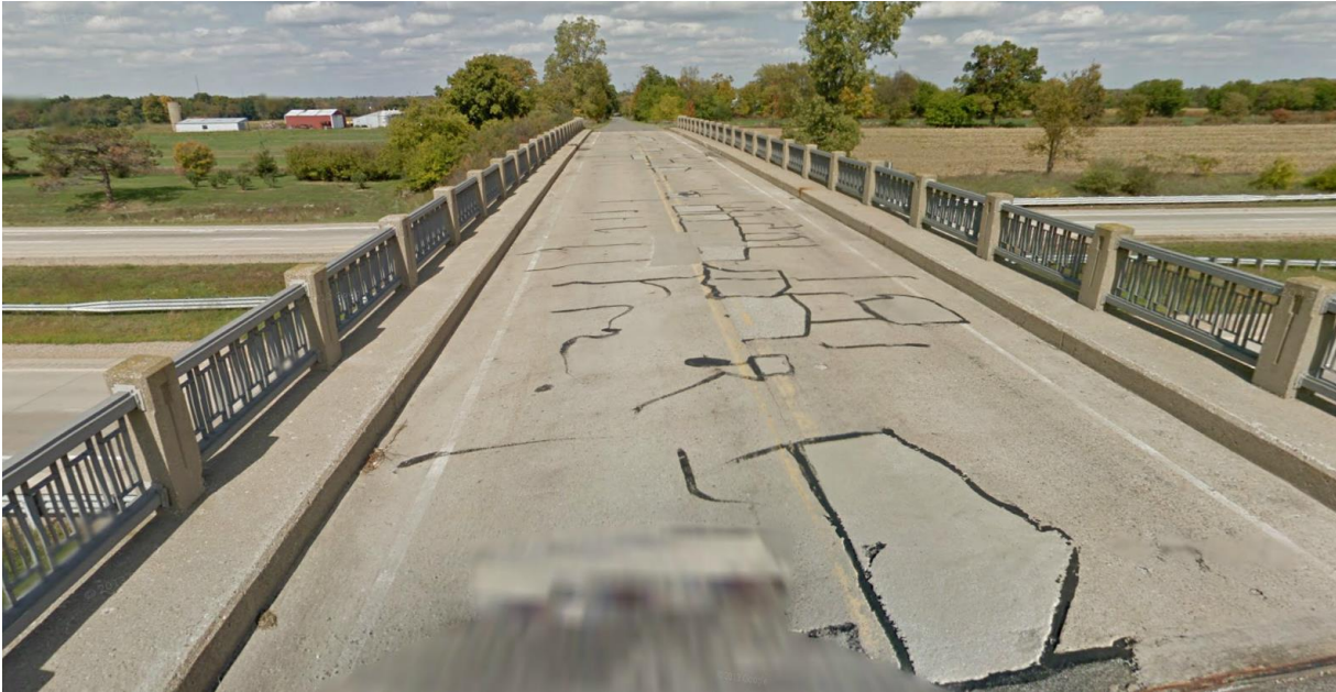
Figure 4-2: Deck Surface for 20 Mile Road Bridge.
