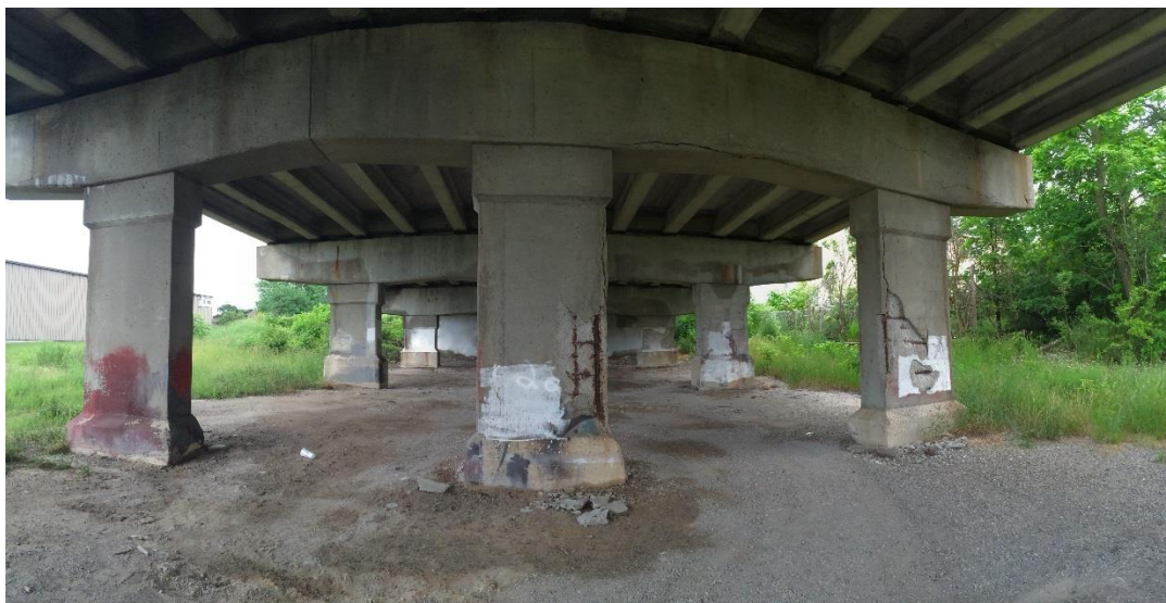
Figure 6-15: Precast Concrete Approach Spans under Franklin Street Bridge.
