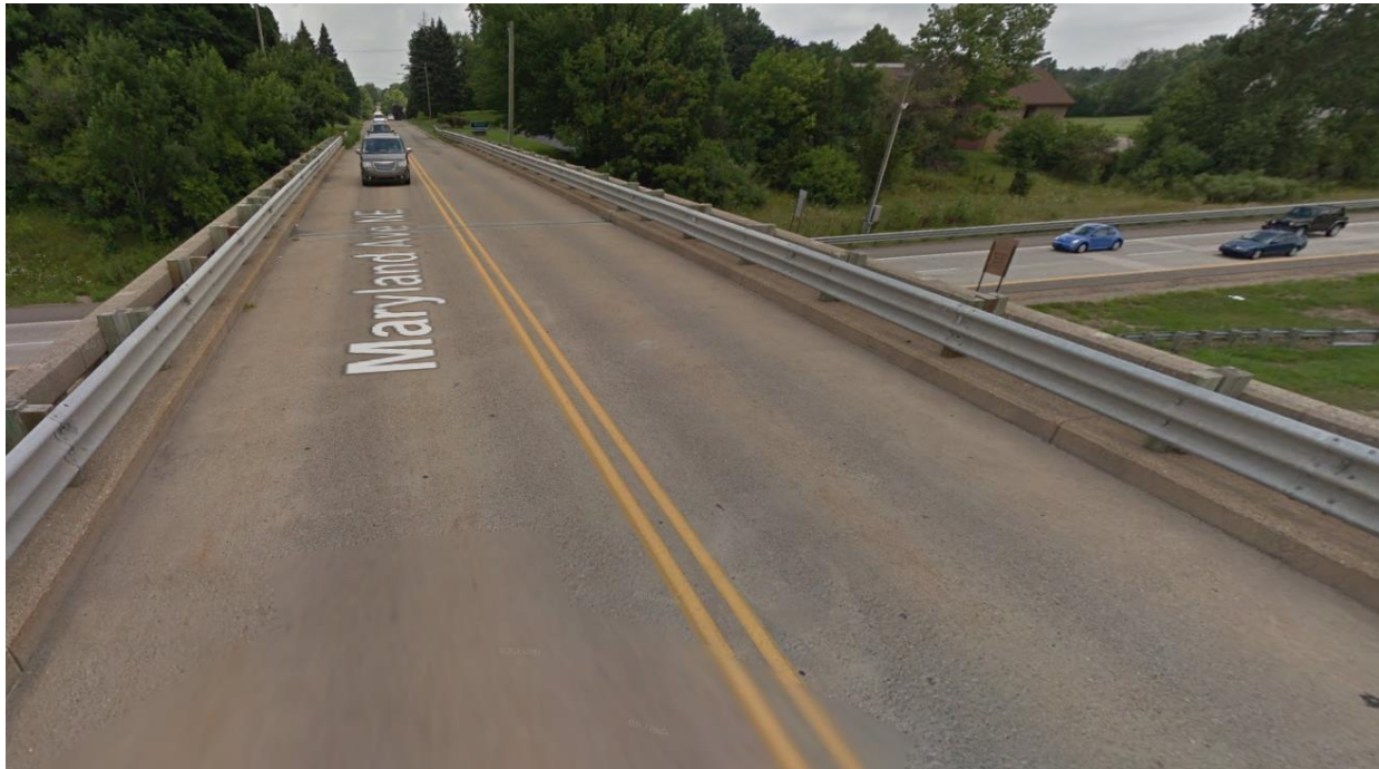
Figure 4-13: Current Condition of the Maryland Avenue Bridge Deck
