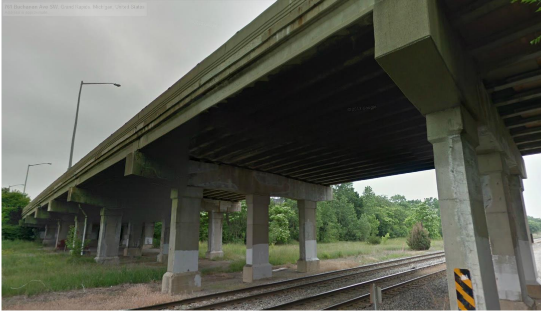
Figure 4-18: Franklin Street Bridge East Side Concrete Beam Approach Structure.
