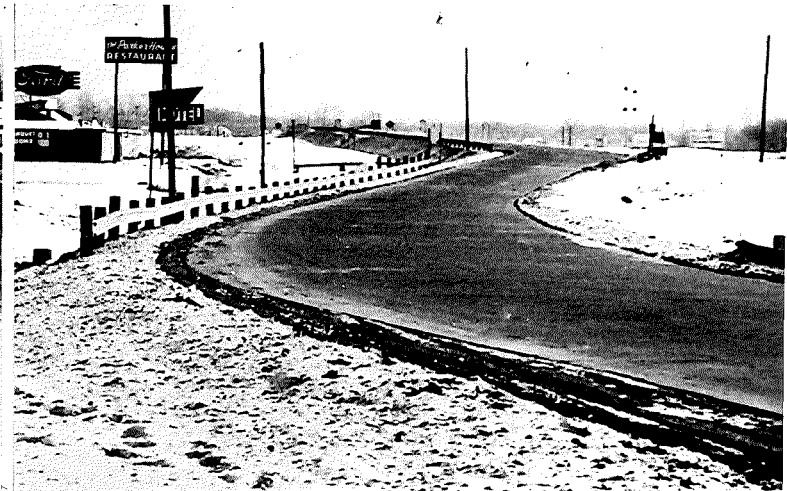
Figure 2. View looking east at I 96 culvert construction area. Sample 63 MR-287 was obtained when permanent guard rail from ramp in background was partially relocated as temporary rail in foreground.
