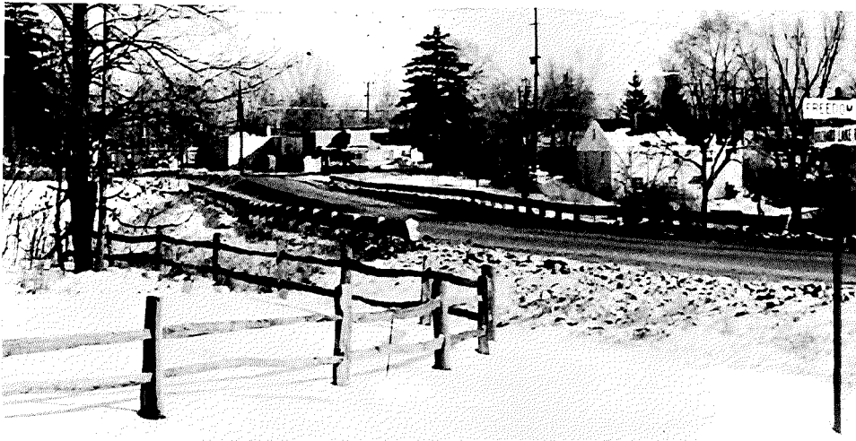
Figure 1. View looking north on Orchard Lake Road, showing guard rail from which decayed posts were removed.
