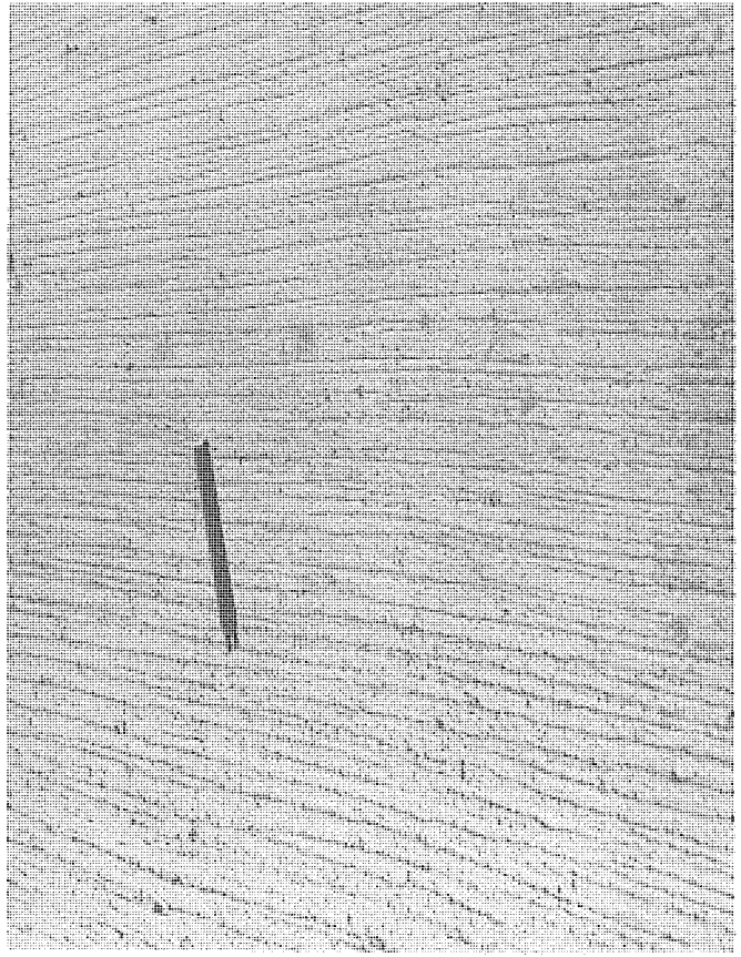
Figure 4. Longitudinal burlap drag finish.
