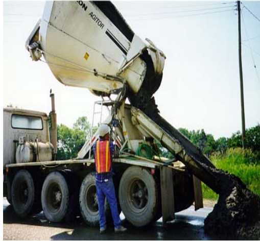
Figure 8. Trucks used for hauling the concrete.
