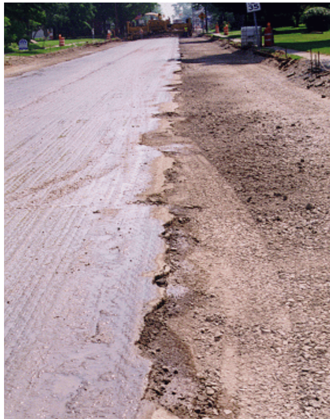
Figure 10. Edge condition after milling.
