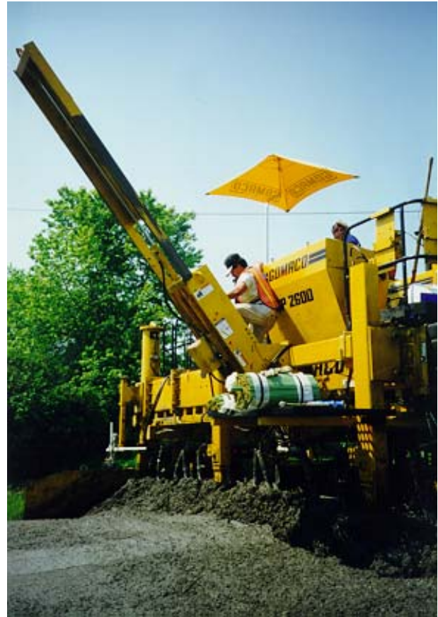
Figure 7. Method for placing tie bars at centerline.
