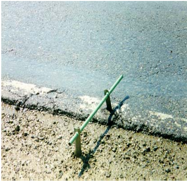
Figure 6. Tie bars setup used at shoulder joints.
