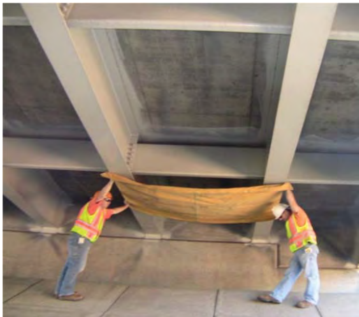
(b) Collecting core from underneath the bridge
