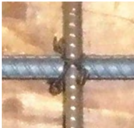
Figure 3-4 Reinforcement tied together with steel wire
