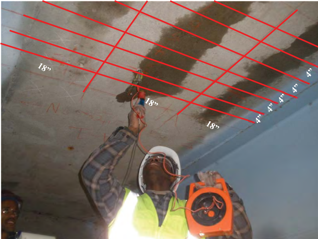
Figure 4-9 Measuring corrosion potential underneath bridge deck with CANIN
