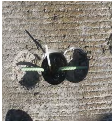
(f) Reinforcement detail in the core hole
