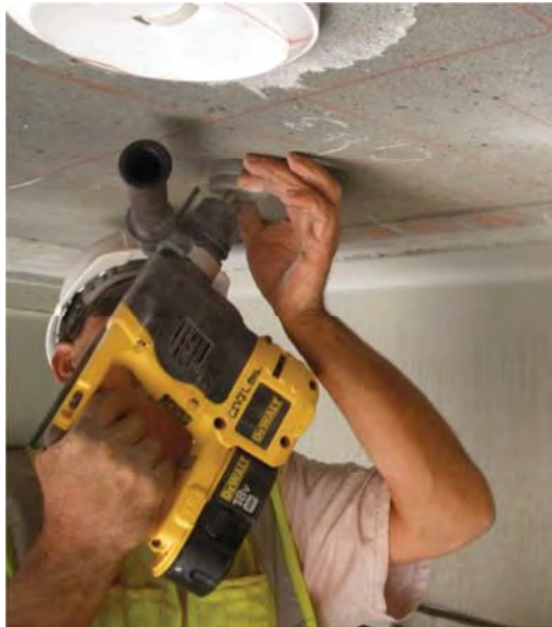
Figure 4-11 Collecting of concrete powder from the bottom deck
