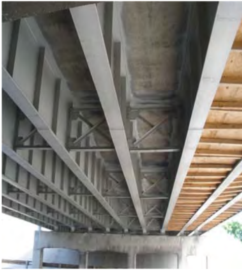
(e) Bottom view of 63174-S05-1 carrying I-75 NB over 14 Mile Road
