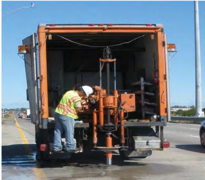
(a) Coring by MDOT personnel
