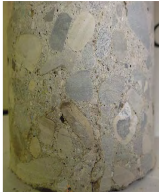
(b) Cracks on the core propagating from bottom surface
