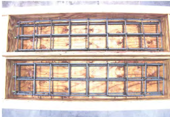
Figure 3-6 Complete forms with the cages
