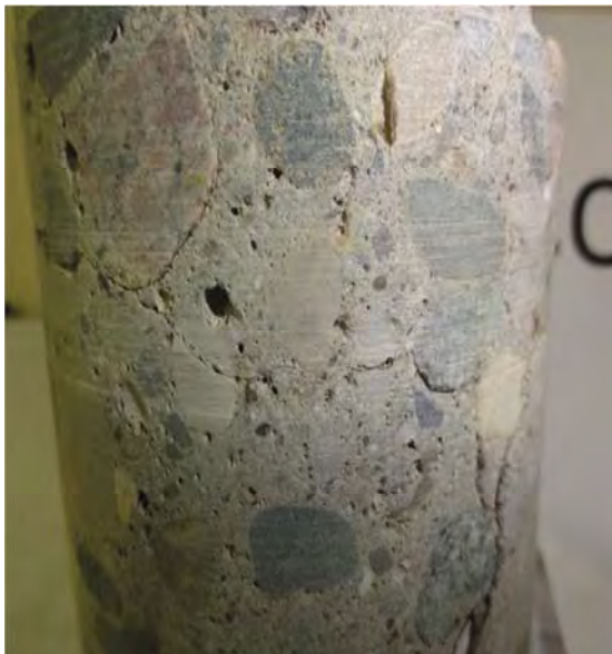
(c) Cracks on core propagating from bottom to mid height
