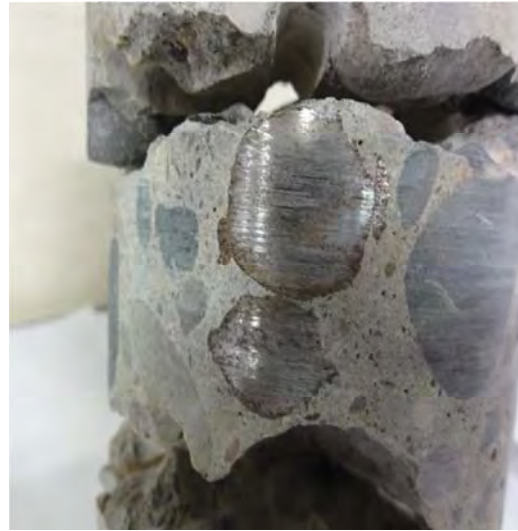
(b) Rust on the reinforcing steel
