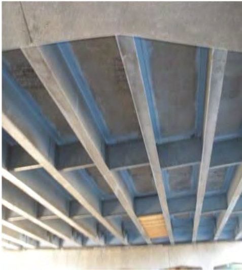
(a) Bottom view of 63022-S02-4 carrying I-96 WB over Milford Road
