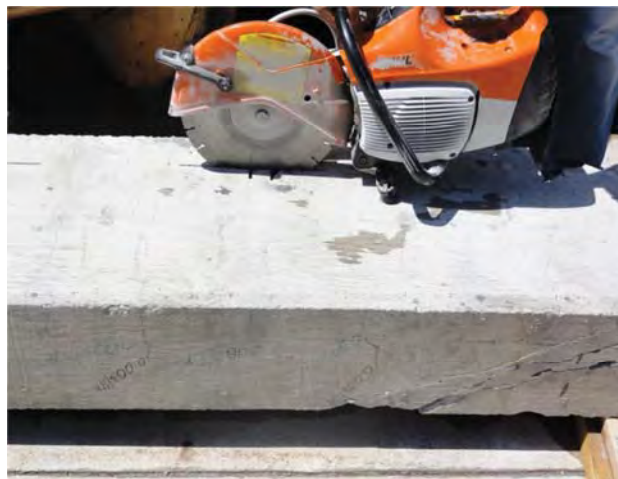
Figure 3-28 Cutting of samples with concrete diamond hand saw
