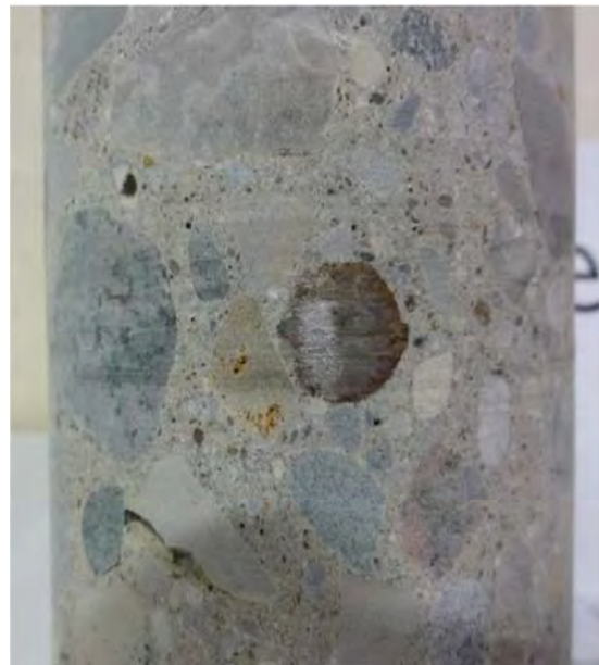
(b) Rust on the reinforcing steel
