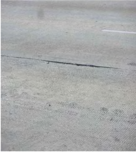
(a) Generally good concrete condition on the wearing surface
