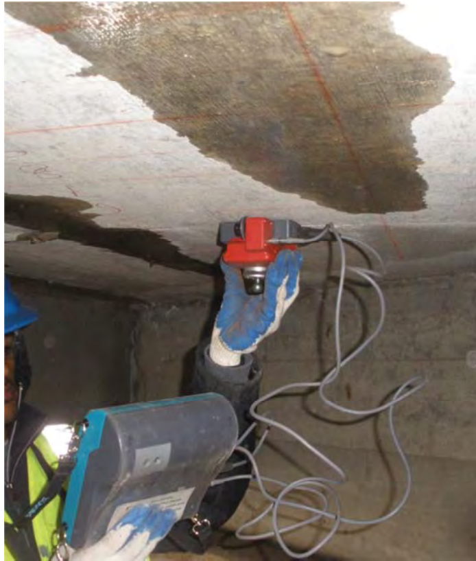
Figure 4-5 Locating a reinforcement bar with Profometer underneath bridge deck
