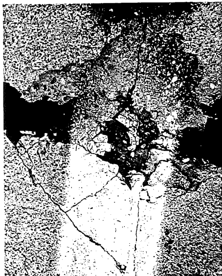
FIGURE 1. D-CRACKING AT A REGULAR EXPANSION JOINT. STATION 102 + 32.
