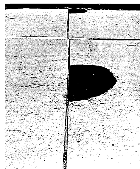
FIGURE 6. NEOPRENE JOINT SHOWING SPALLING AS OF AUGUST 3, 1953.
