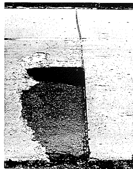
FIGURE 5. BAD DISINTEGRATION AT NEOPRENE JOINT WHICH DEVELOPED MOSTLY DURING LAST WINTER AND IS CONTINUING AT THE PRESENT TIME. STATION 131 + 29.
