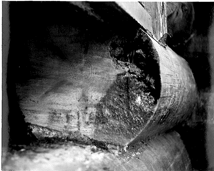
Figure 8. Log adjacent to west end of section removed.
