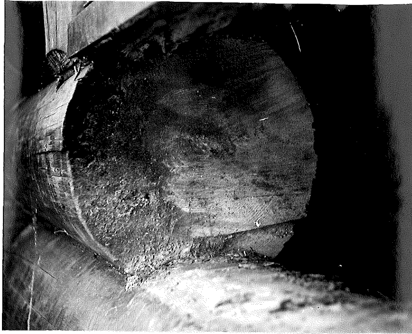
Figure 7. Log adjacent to east end of section removed.
