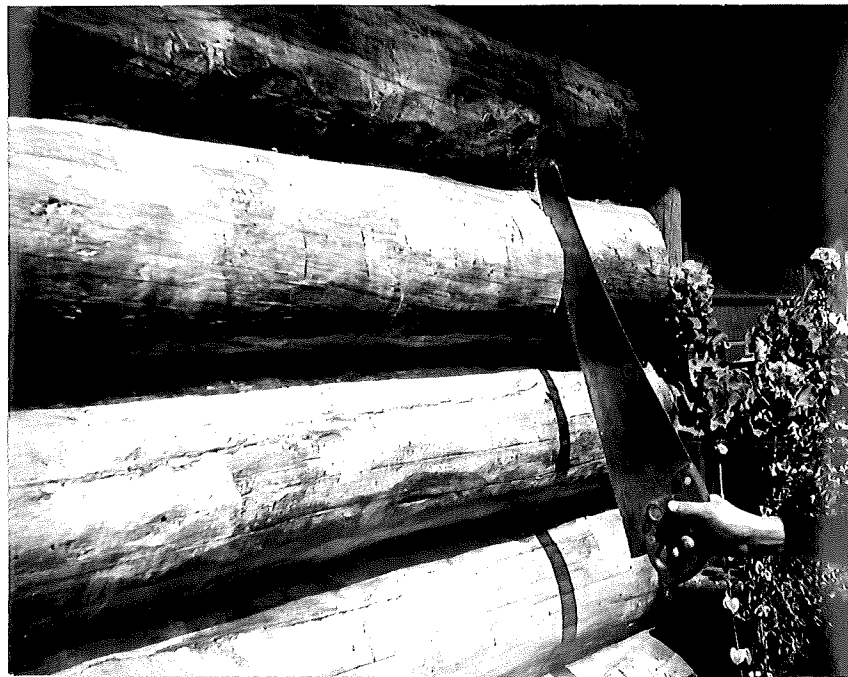
Figure 4. Removing sample at point shown in Figure 3.
