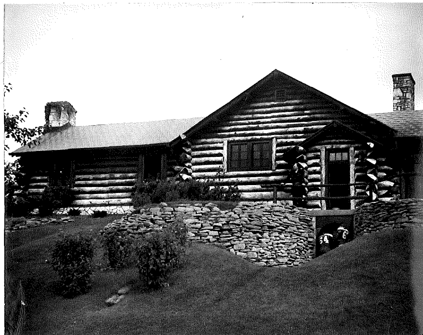
Figure 2. Rear view, south wall.
