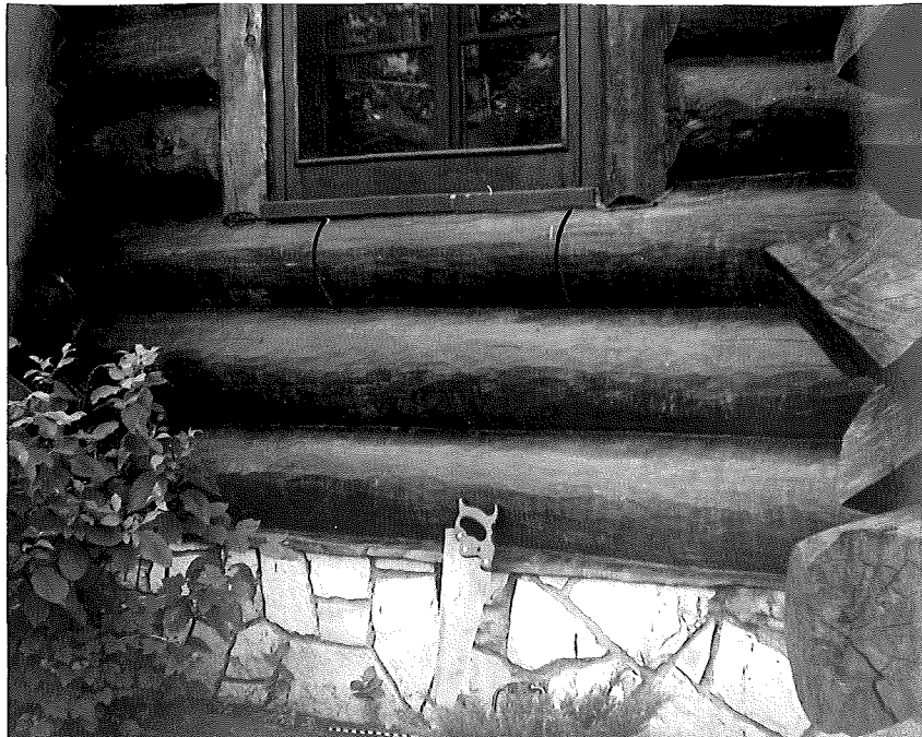
Figure 6. Portion of north wall showing point at which section of log was removed for study at Michigan State College.
