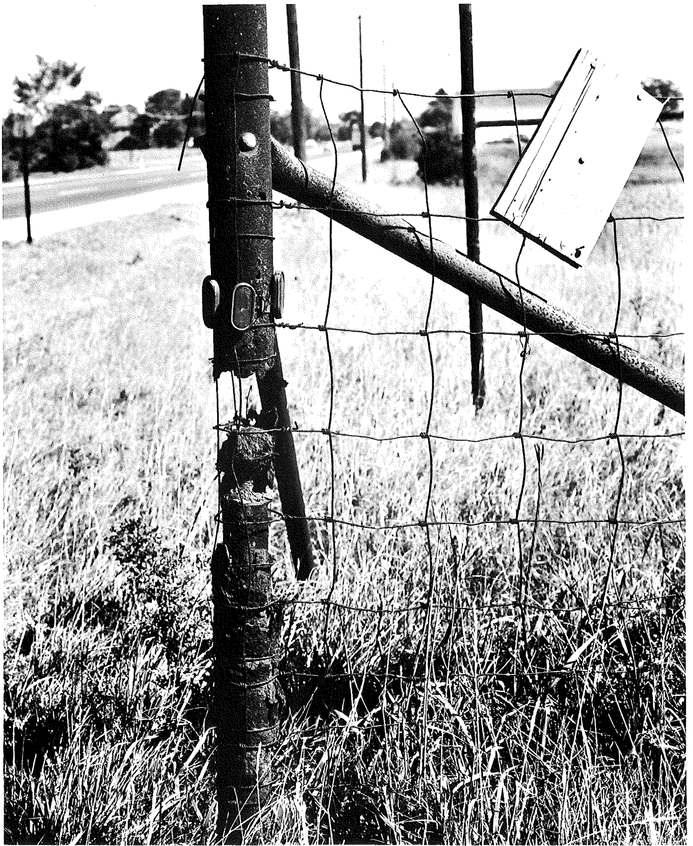
Figure 10. Age: 24 years. South-east corner of East Grand River Road (formerly US 16) and Bauer Road between Brighton and Howell. Corner pipe post corroded through about 2-1/2 ft above ground level, upper portion held up by brace posts.
